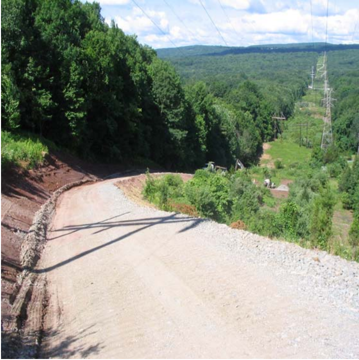
Old Lane Rd (Hamden): Access road construction continues.
