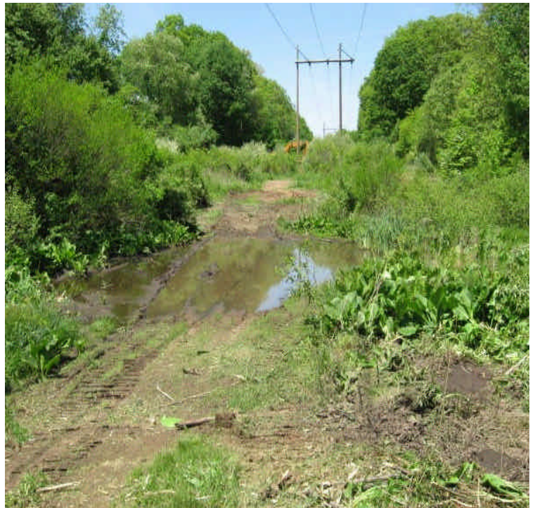
New clearing and small pool crossing off Pond Hill Rd. Controls and approved crossing method are needed.
