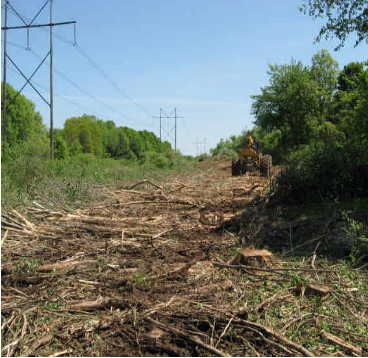
Wetland crossing using timber/corduroy off Powers Road.
