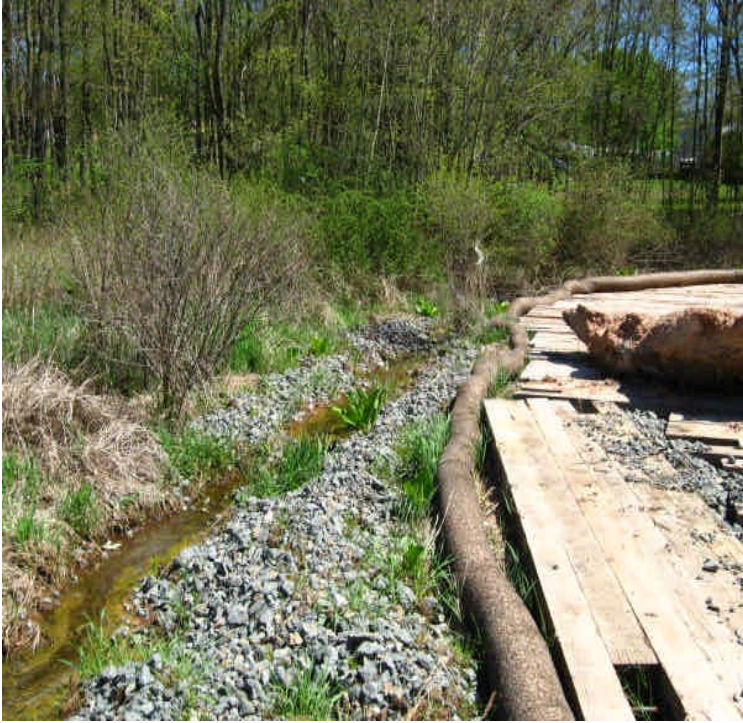
Controls and timber mats off Powers Road.
