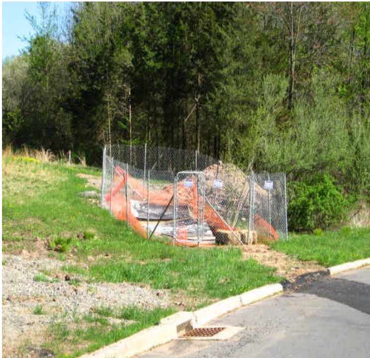
An area of adjacent exposed soil and leftover fill is located in the overhead ROW off Old Farms Rd. Extra material should be removed or controlled and the disturbed area should be stabilized.
