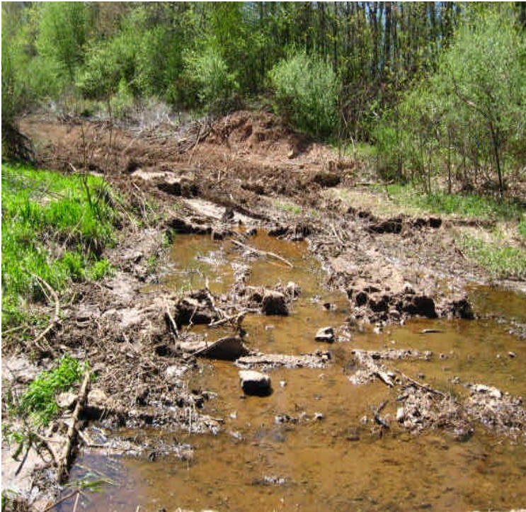
Wetland crossing off Williams Rd. Controls are needed to contain the disturbed soil and prevent run-off to the wetland.
