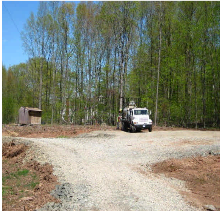
Crews were preparing to hydroseed exposed soil north of Stony Brook Road.
