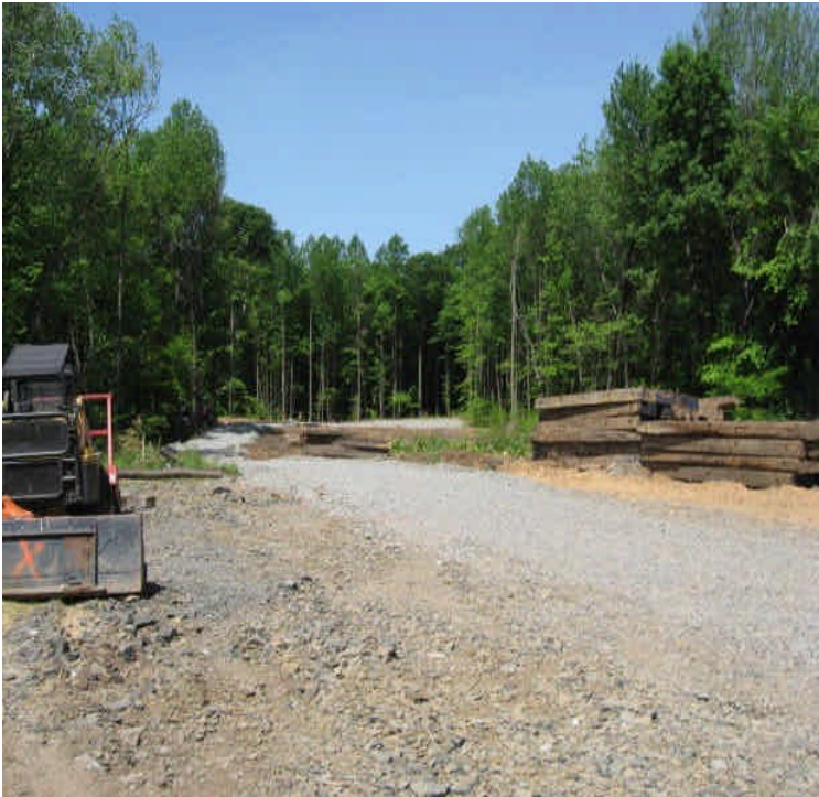
ROW access road installed moving west from the contractor receiving yard.
