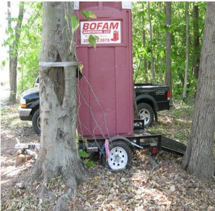
Portable sanitary facility located immediately at the wetland boundary in the watershed protection area. Note pink & blue wetland flagging. Vehicles and facility should be relocated.
