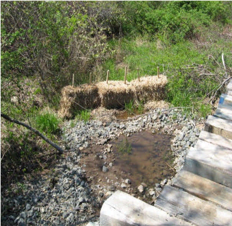
Stormwater controls remain adjacent to the timber mat crossing off Rte 17. Clear water was flowing off site.
