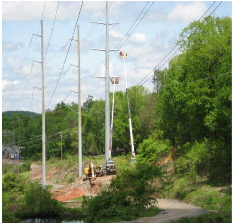
Line installation continues near East Meriden SS.
