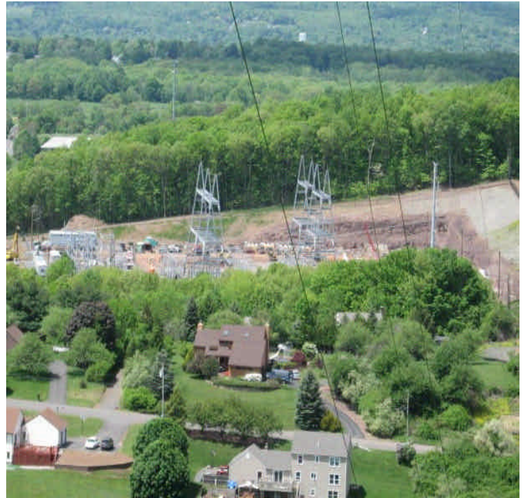
Looking west from Beseck Mountain towards the construction at Beseck SS
