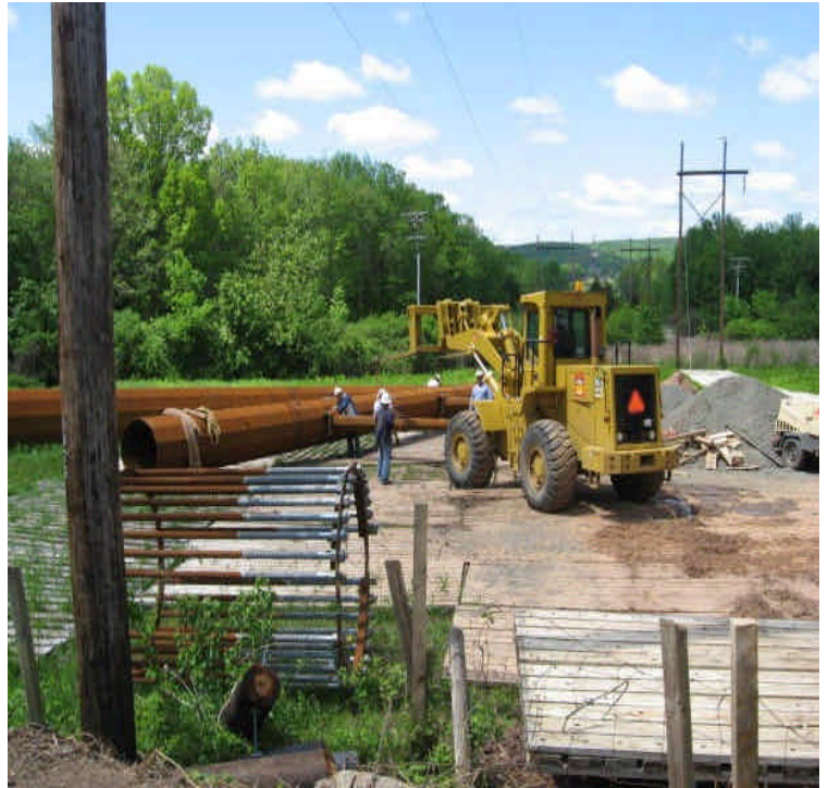
Structure work noted off Cherry Hill Rd.
