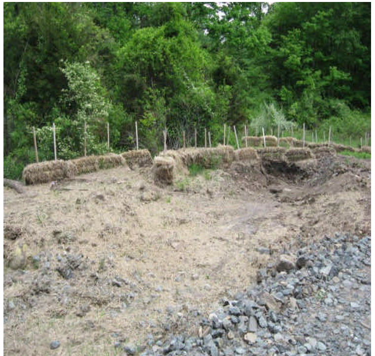
Hydroseed and haybales remain in work areas west of Powder Hill in an effort to restore the area.
