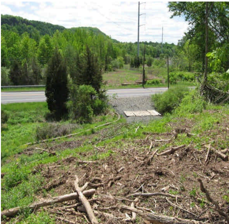
Site access north of East Main Street. Controls/filter socks were installed.
