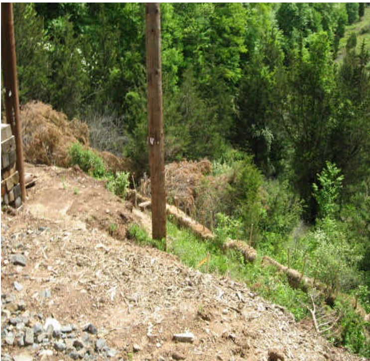
Haybale line at the final pad upgradient from Ball Brook off Black Walnut Dr.
