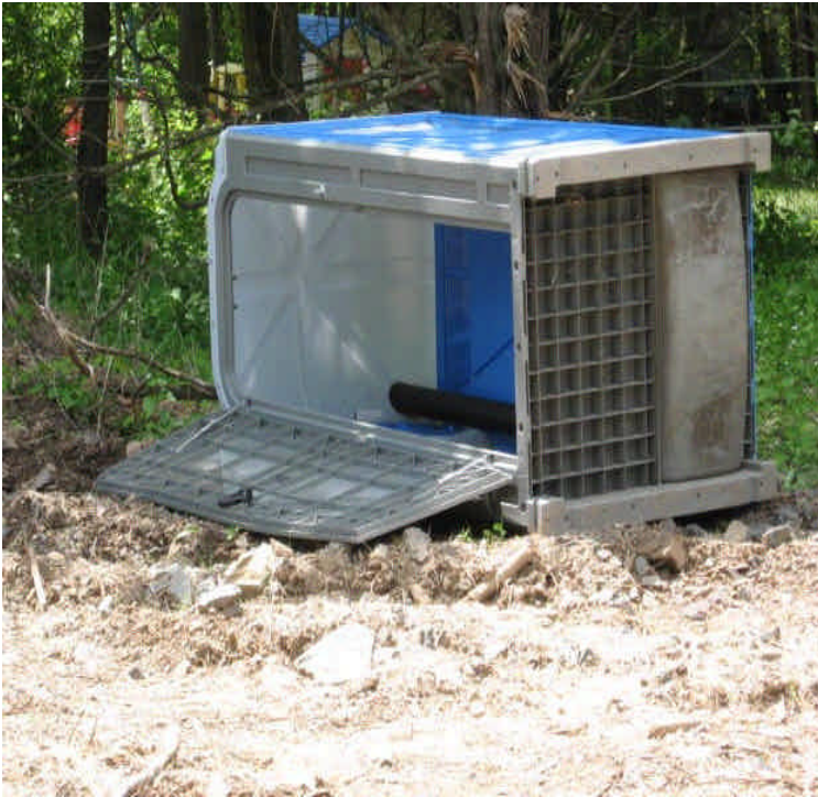
A portable sanitary facility west of Powder Hill Rd. has tipped over. This should be righted and secured.
