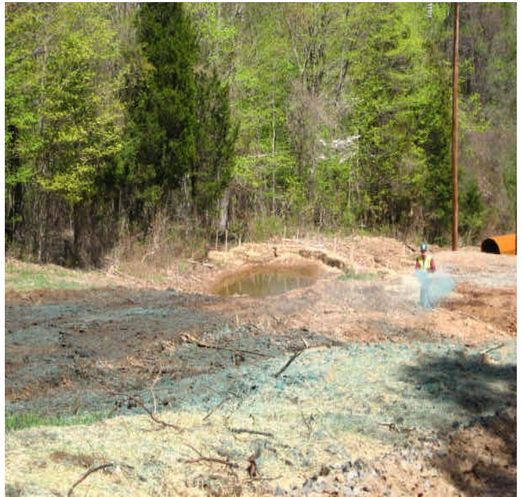
Hydroseeding was noted west of Powder Hill in an effort to restore the area.
