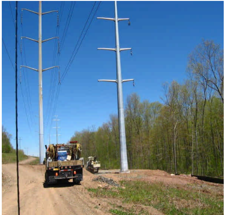
Crews were placing pulleys for wire/line installation north of Beseck SS.
