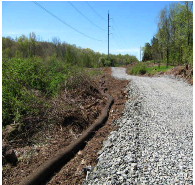
New access road and controls off East Main Street looking south.
