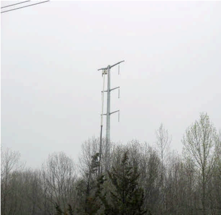
Pole work east of Beseck SS. off Valley View Drive.
