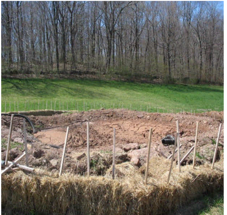
Slurry/dewatering containment area in place just north of Beseck SS.
