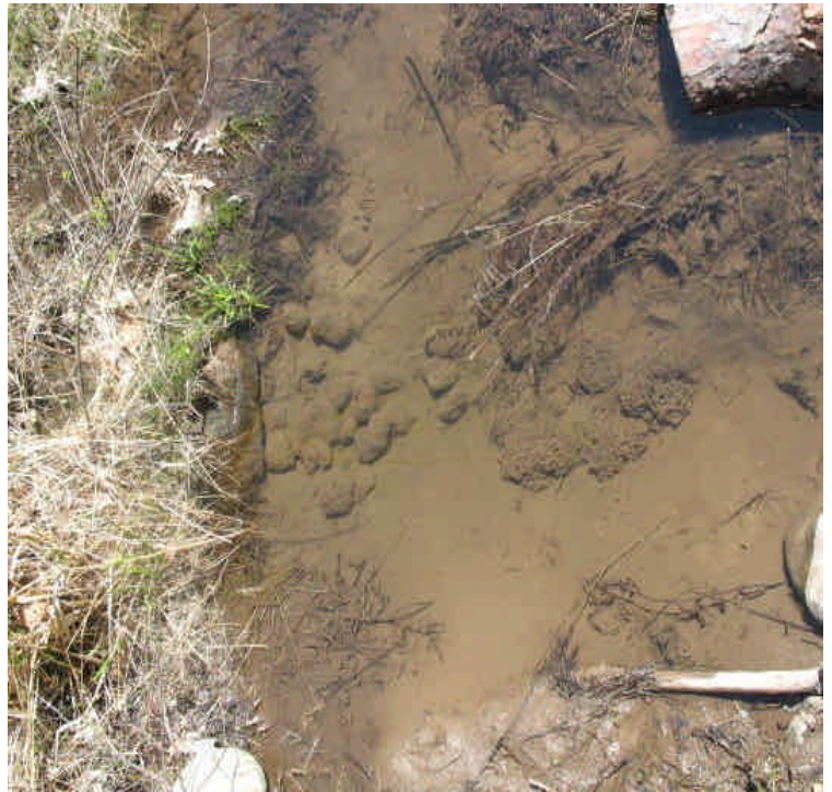
Amphibian egg masses were noted in the ponded water adjacent to a timber mat crossing off Johnson Ln. Slight sedimentation resulted from recent heavy rain. Continue to prevent turbidity and sedimentation here to the extent possible.
