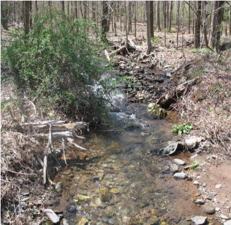
Wetland and stream crossing off Foot Hills Rd. Mats were in place and turbid run-off was not noted.
