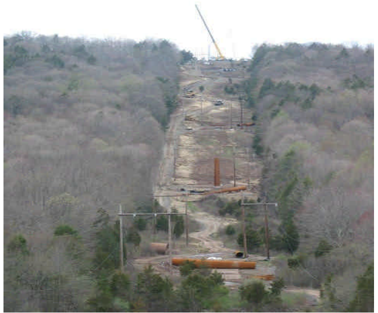
Looking west from Powder Hill Road. Pole installation is underway.
