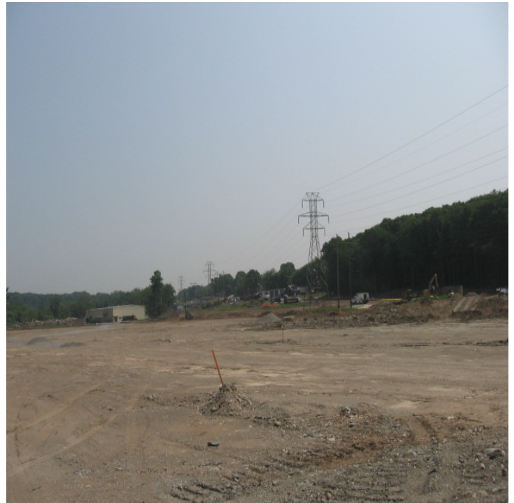
Overall view of the substation site. Grading and foundation construction continues.
