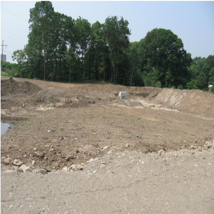
Detention basin construction continues at the southeastern portion of the site.
