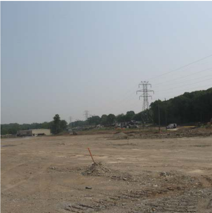
Grading continues throughout the site.
