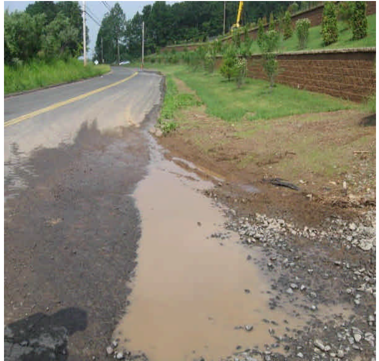
View of eastern site exit along Carpenter Lane. Haybales were removed and not replaced at the corner of this area and turbid run-off from the storm was flowing off site.
