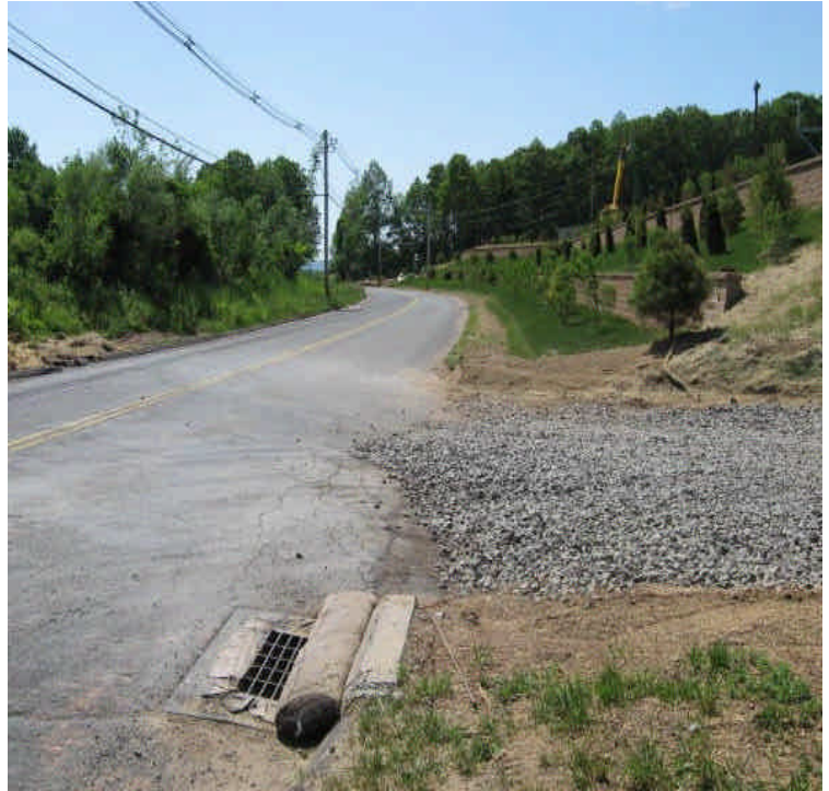
View of eastern site exit. The silt fence was removed along Carpenter Lane and haybales were removed from the exit. Apply seed to any exposed soil resulting from the removal.
