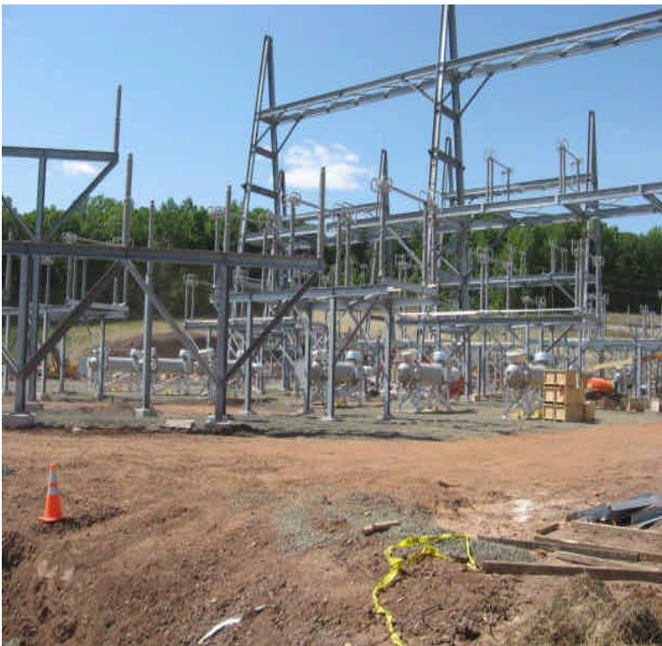
View of the entire site from the southeast corner looking north. Stone is being spread at completed areas for further stabilization.
