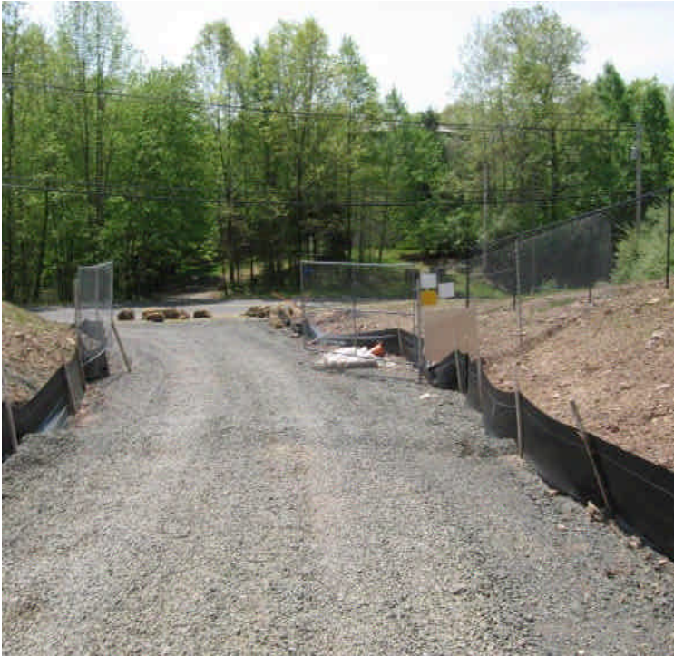
Site entrance off Carpenter Lane is at final grade. Stone base and stone check dams remain in place
