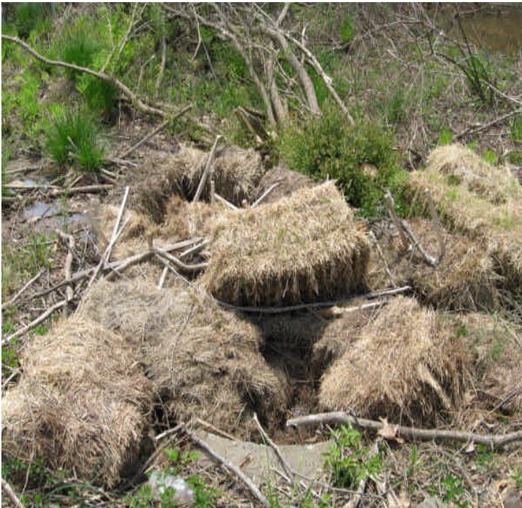
Storm drain outlet across Carpenter Lane has clear water flowing through the haybales.
