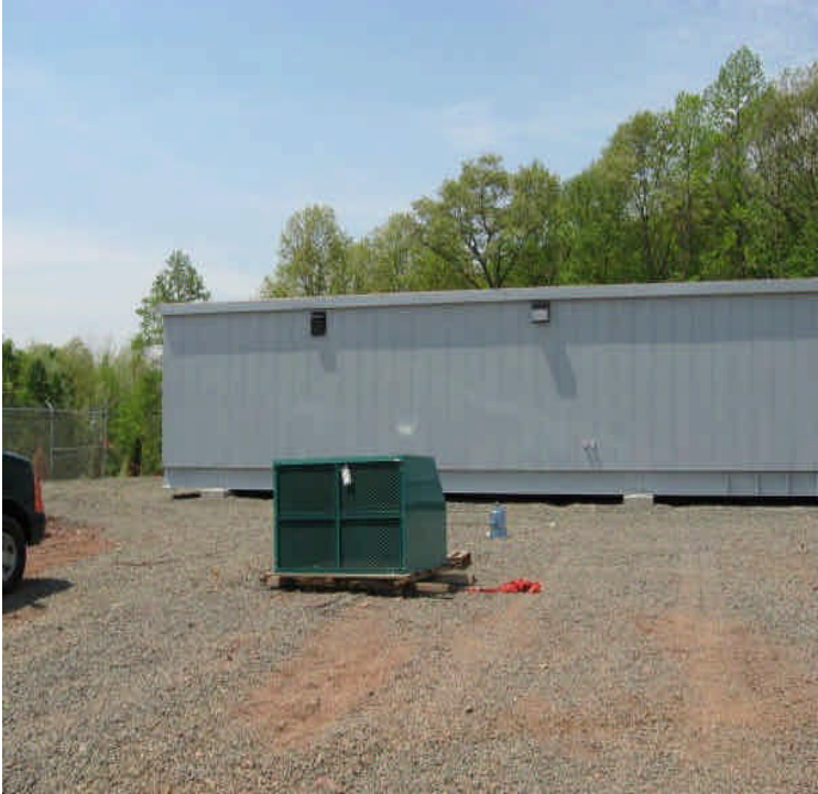
A new building was in place in the southwestern side of the site. Stone base was also applied to stabilize soil.
