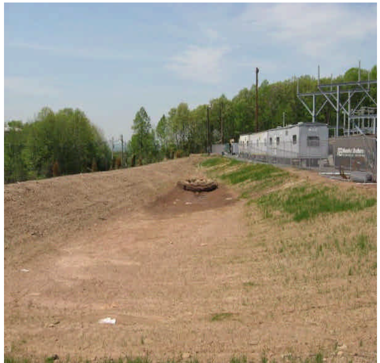
Haybales and controls remain in place at the inlet of the detention basin. Sediment from stormwater run-off has settled in the basin. Consider adding more seed here for further stabilization.
