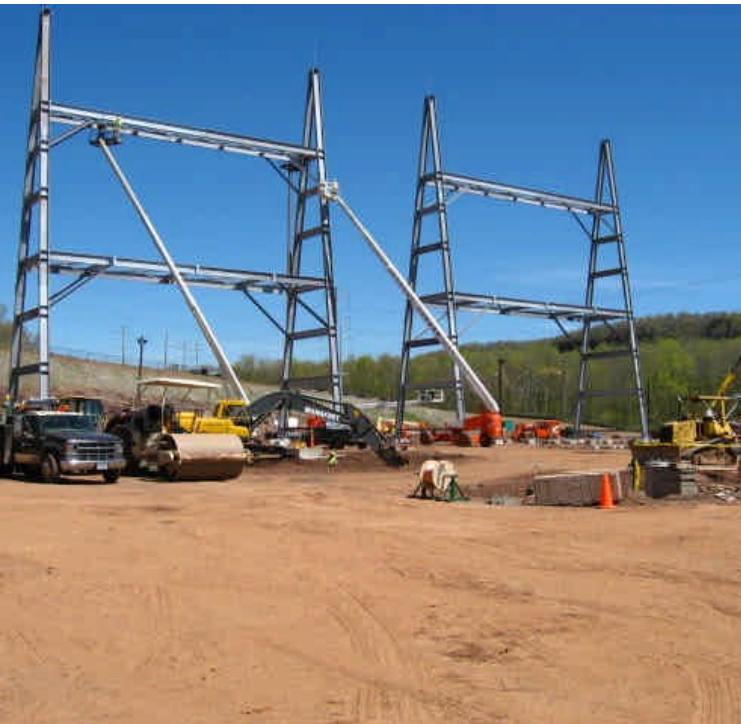
View of the site and some of the structures being installed.
