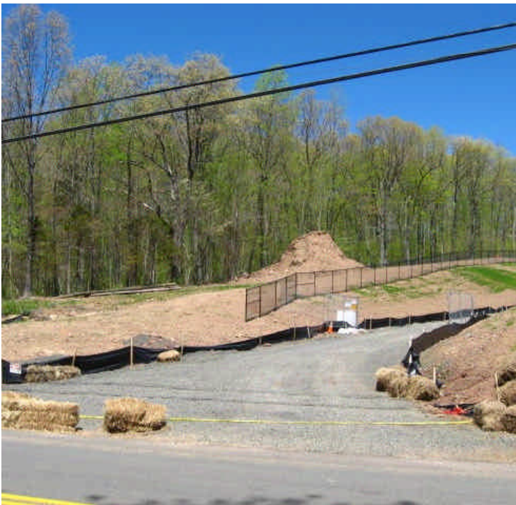
Site entrance off Carpenter Lane is well controlled. Replace controls across the drive when feasible.
