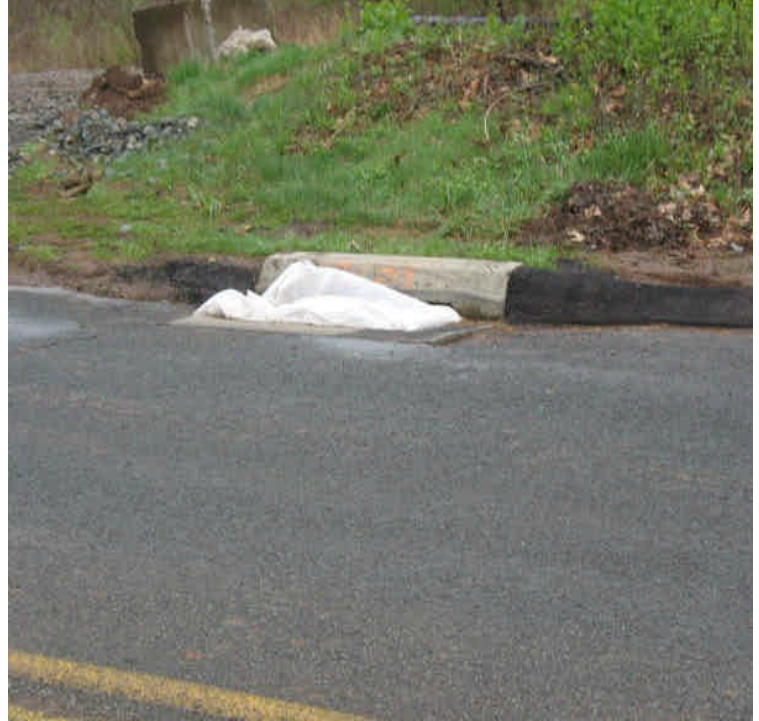
The catch basin liners along Carpenter Lane have been replaced.
