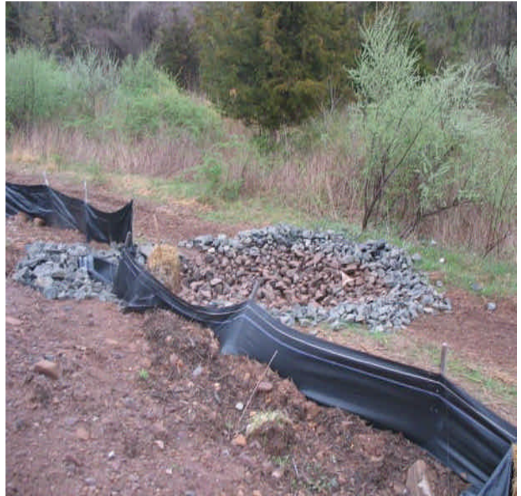
View of the culvert and sediment trap under the access road to the ROW. This control works well for smaller storms but needs reinforcement during the larger rain events.
