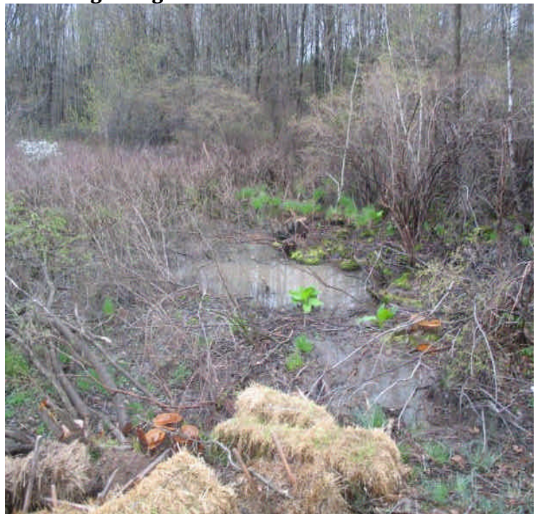
Turbid water was observed leaving the haybales and ponding in the wetlands. Evaluate whether the amount of sediment accumulation justifies the minor disturbance needed to remove it, once the water subsides.
