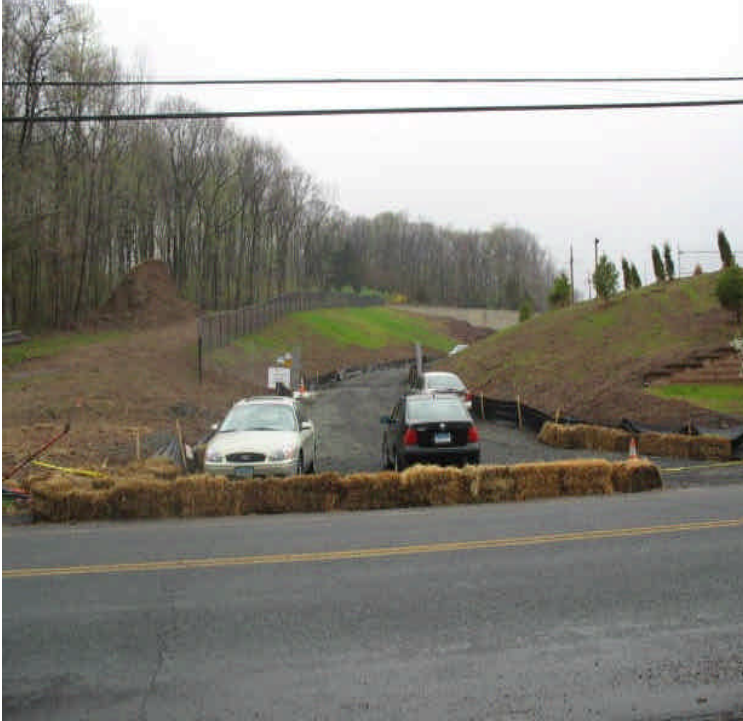
Site entrance off Carpenter Lane is well controlled; the area is being used for temporary parking of personal vehicles.
