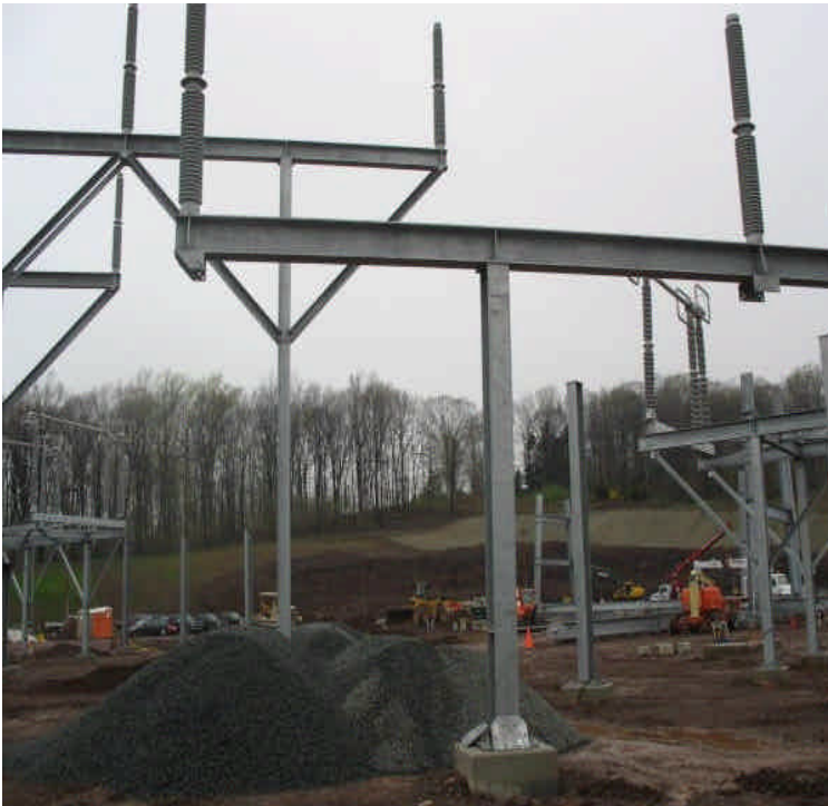
View of the entire site from the southeast corner looking north.
