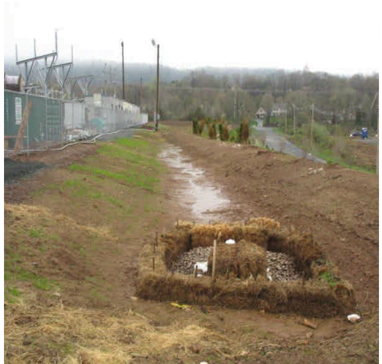
Haybales and controls remain in place at the inlet of the detention basin. Sediment from the stormwater run-off has settled in the basin.
