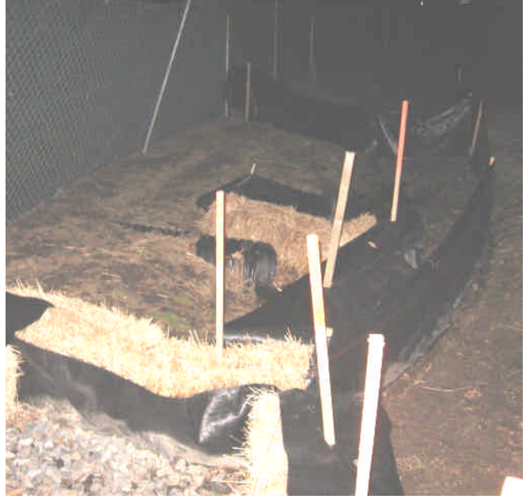
Both photo are of the Sherwood Island lay-down yard. Left: The entire yard has been lined with fabric and covered with a layer of stone. This will reduce mud and tracking as well as allow for simplified clean-up or restoration. Right: The only stormwater discharge point from the site has been adequately protected with erosion controls.
