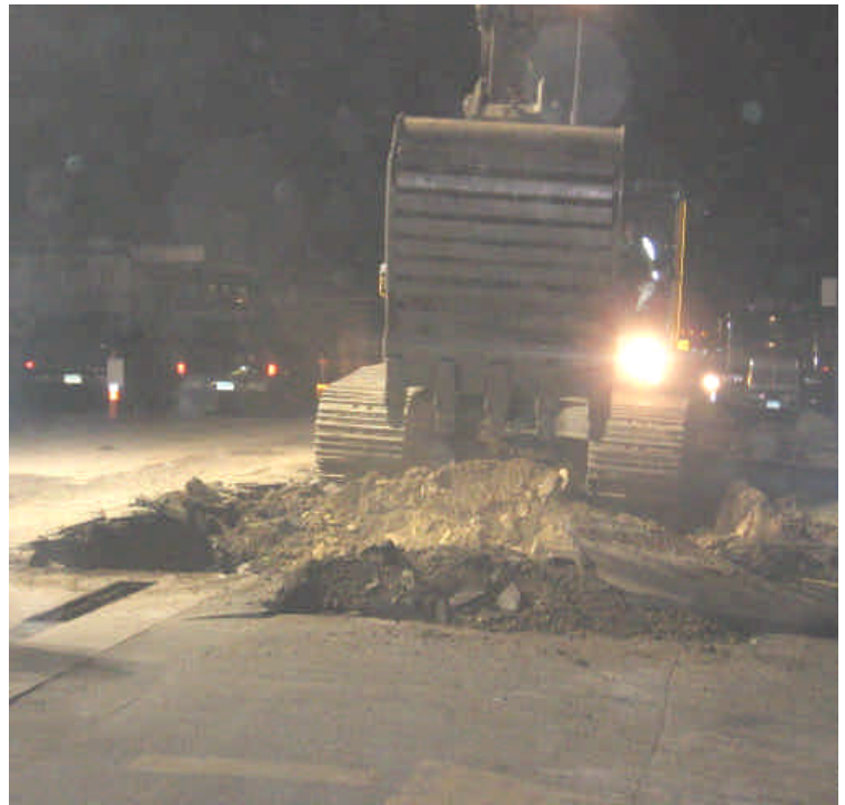
Excavation activities for Vault #20 were initiated during this week's inspection.
