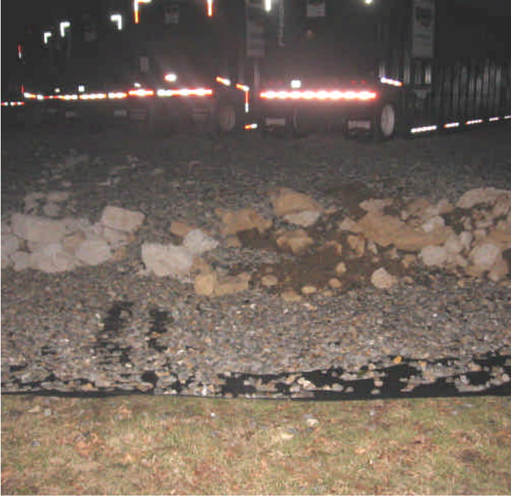
Both photo are of the Sherwood Island lay-down yard. Left: The entire yard has been lined with fabric and covered with a layer of stone. This will reduce mud and tracking as well as allow for simplified clean-up or restoration. Right: The only stormwater discharge point from the site has been adequately protected with erosion controls.
