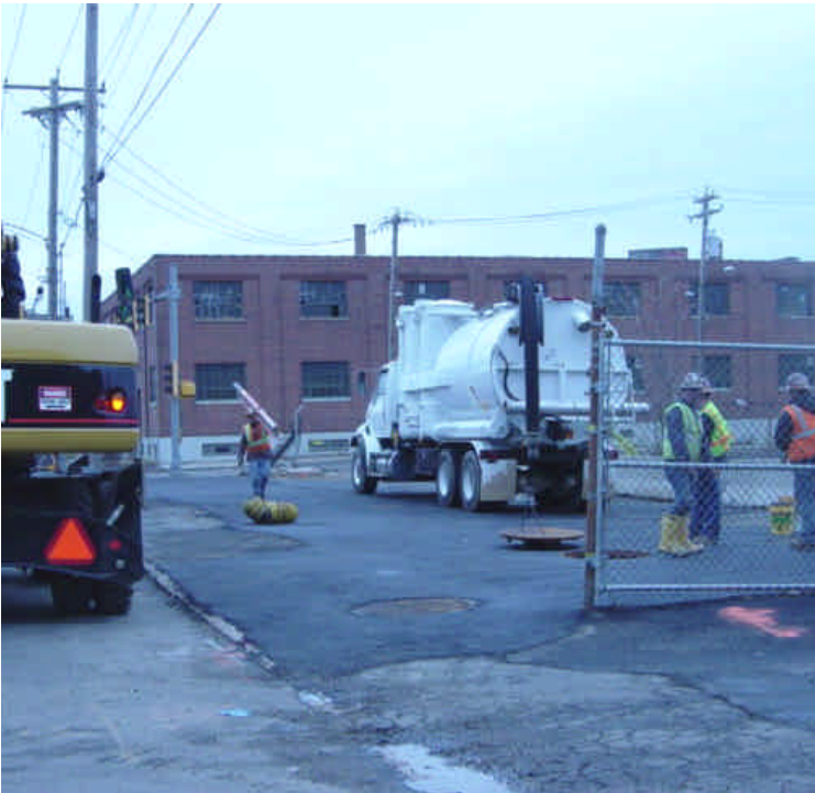
Trenching activities at the corner of Bostwick Ave. and Railroad Ave.
