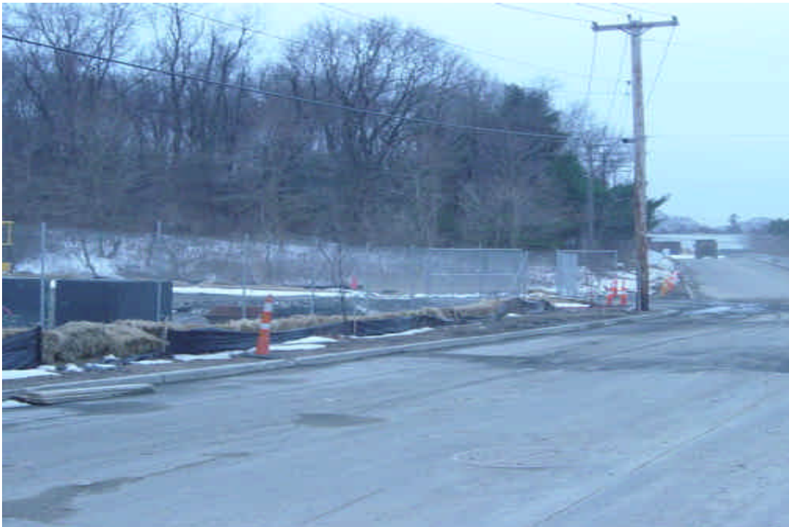
Minor tracking was evident along the roadway at the entrance to the Milford lay-down yard.
