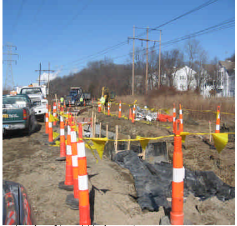
View of trenching activities from station #1061 to 1063.
