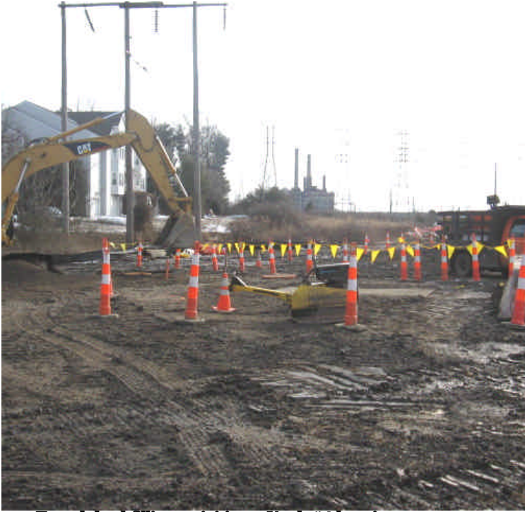
Trench backfilling activities at Vault #4 location.
