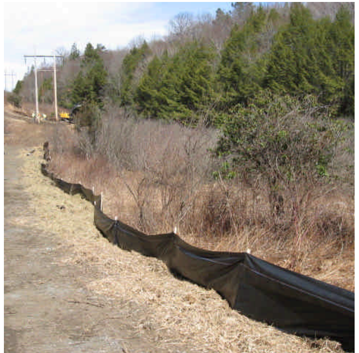
Cow Path Lane: Mulch was in place along the disturbed edges of the access road.
