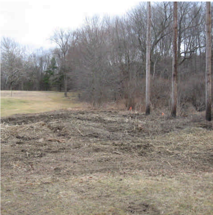
Oak Lane Country Club: The wetland has been cleared for crane pad construction.
