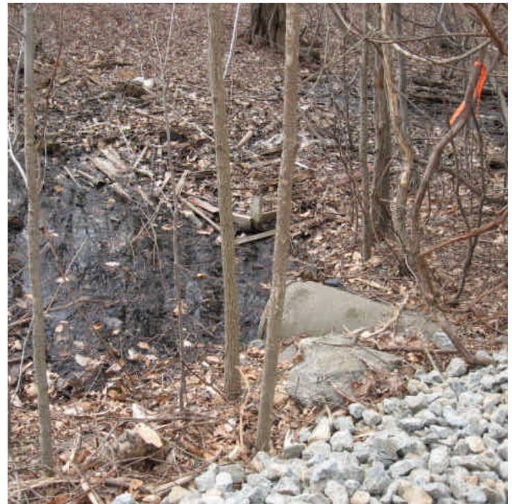
East Rutland Rd: View of the pre-existing culvert crossing
