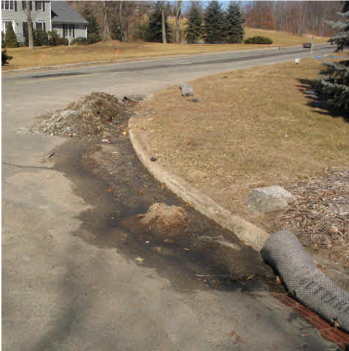
Old Lane Rd (Hamden): Snow/sediment remains along the roadway from plowing activities. Gutter buddies remain at the curb inlets.
