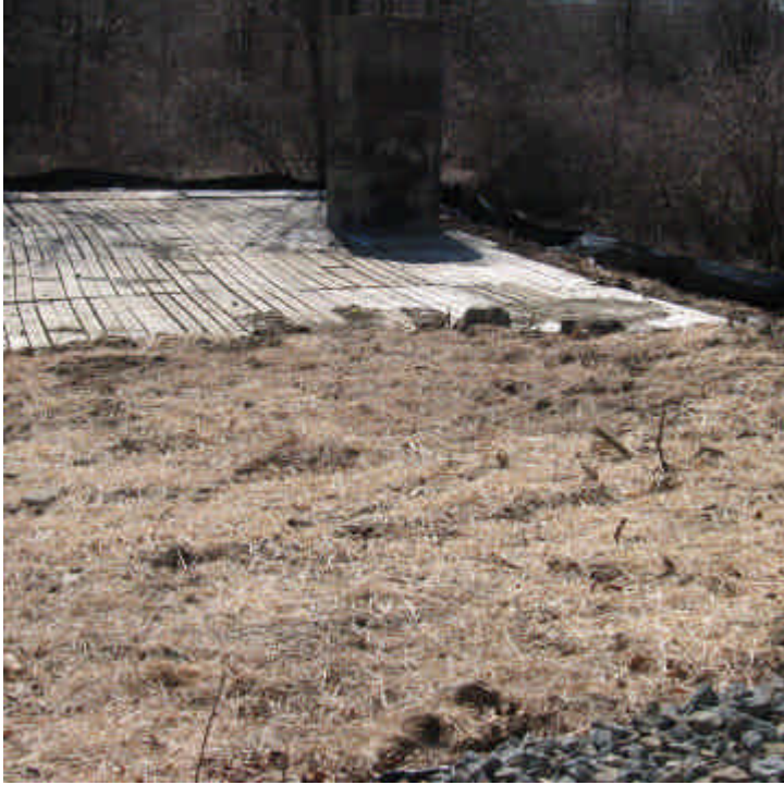
Route 121 (Milford): Erosion controls remain intact at the wetland here. Mulch was is in place along the disturbed slopes.
