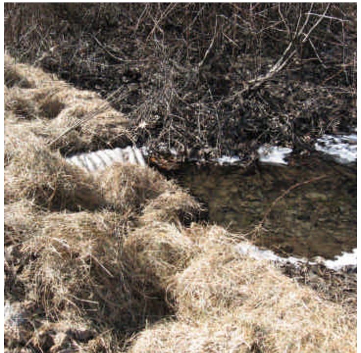
Treat Lane: Haybales were installed at the stream in an effort to further prevent sedimentation.
