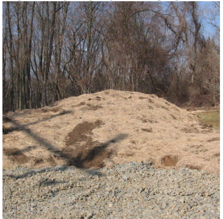
Hay mulch has been applied to the disturbed areas here (Woodruff Rd.)
