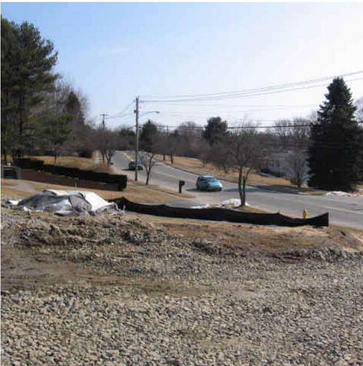
View of the foundation installed within the ROW off Woodruff Rd.
