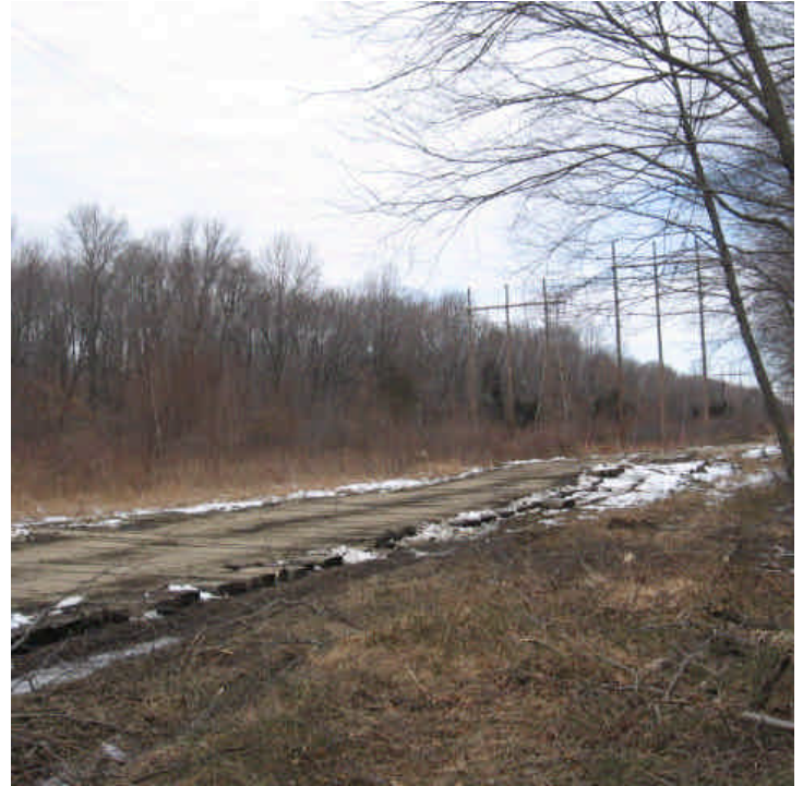
Additional timber mats have been placed along the access road to support equipment here (Pease Road).
