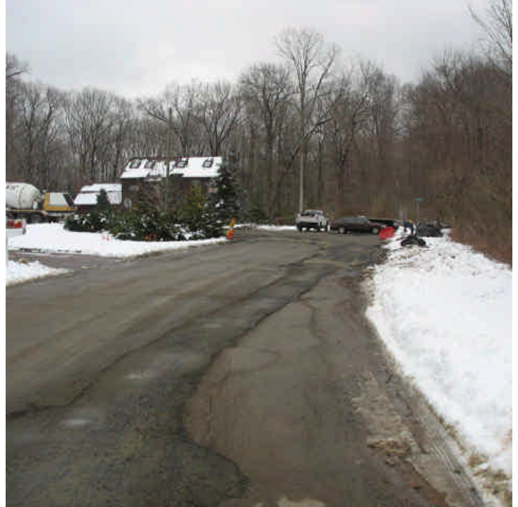
An additional view of the 115-kV work within Old Lane Road.
