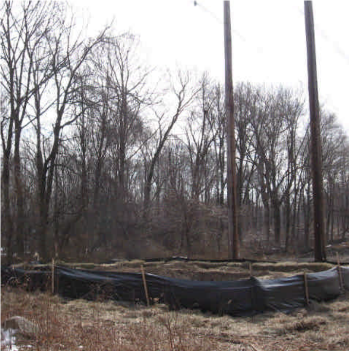
Dewatering controls were installed proactively within the ROW here (Pease Road).
