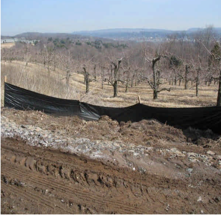
Sediment accumulation was noted near some of the controls within the apple orchard off Mansion Rd. Pull back sediment to reduce stress on the controls when needed.
