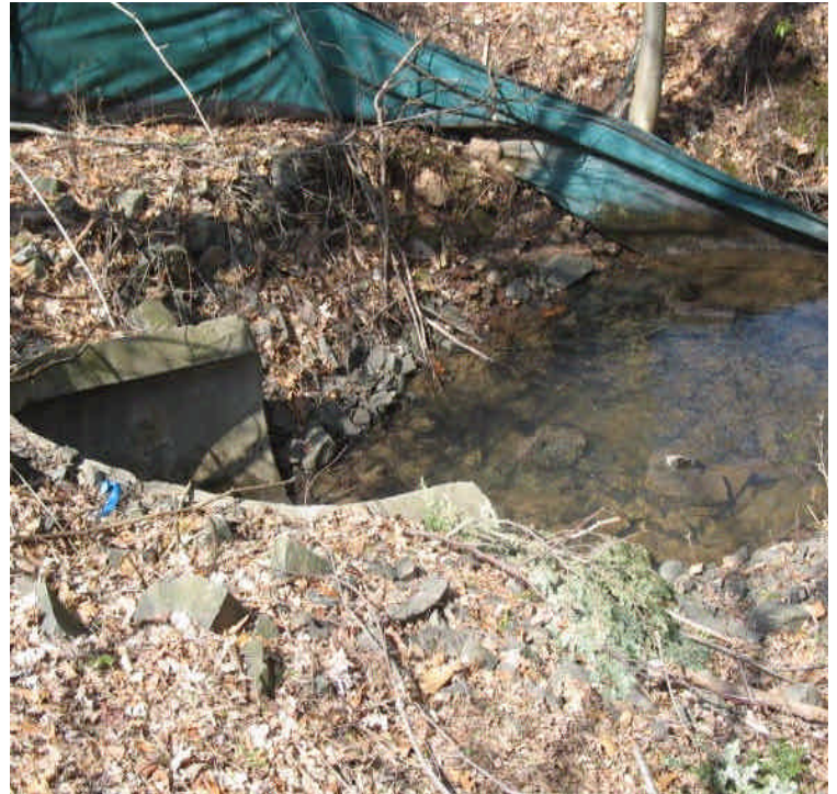
View of one of the receiving wetlands/inlets along Old Farms Rd. Turbidity related to the project was not evident in the wetland at this time. However, issues have been noted during past thaw periods. Continue to monitor.
