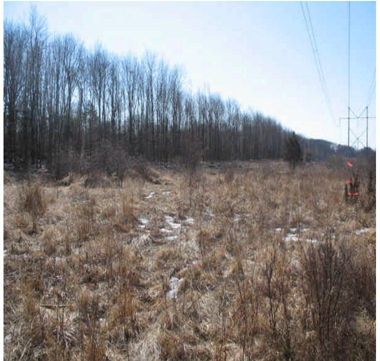
View of vegetation retained following low impact clearing south of Carpenter Ln and Beseck SS. The remaining vegetation will stabilize soils within the wetland.
