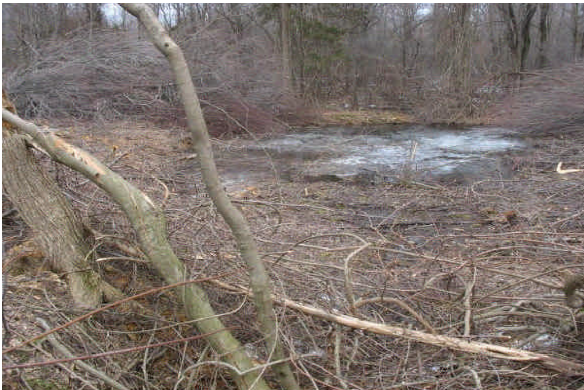
View of a wetland within the ROW, which was bypassed by accessing the ROW from two different points. Equipment remained outside of wetlands to minimize direct impacts.
