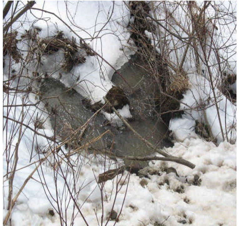
Wetland crossing off Powder Hill Road. Slightly turbid water was observed flowing from the stone crossing despite controls.
