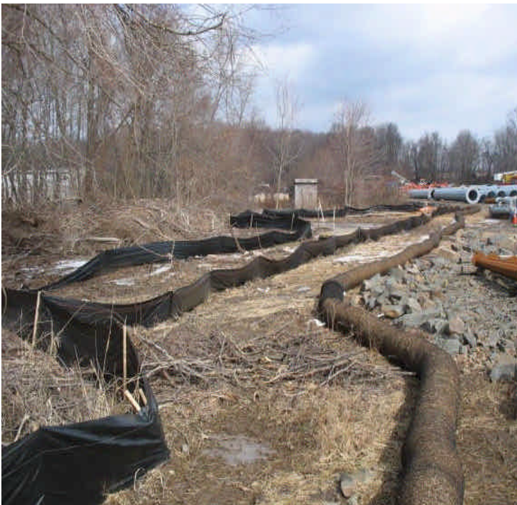
Additional controls remain in place adjacent to wetlands to filter/contain turbid run-off leaving the site.
