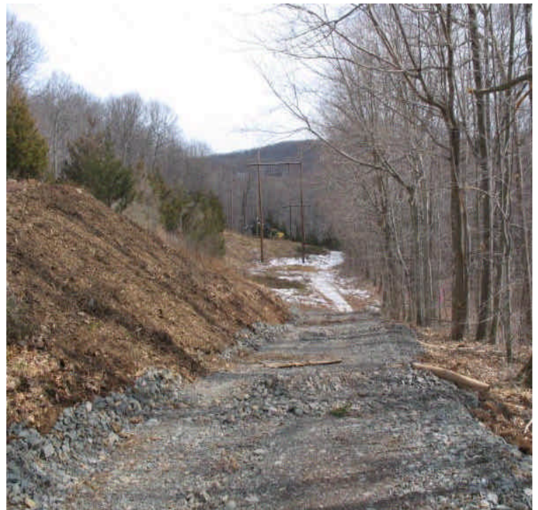
Access road and pad construction continue off Black Walnut Dr.
