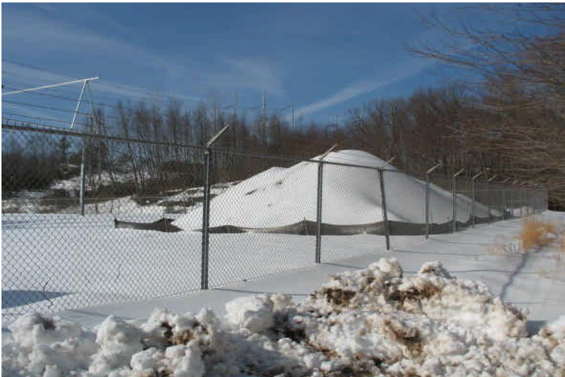
Soil stockpile to be removed. Controls are intact and sediment issues have not been observed.
