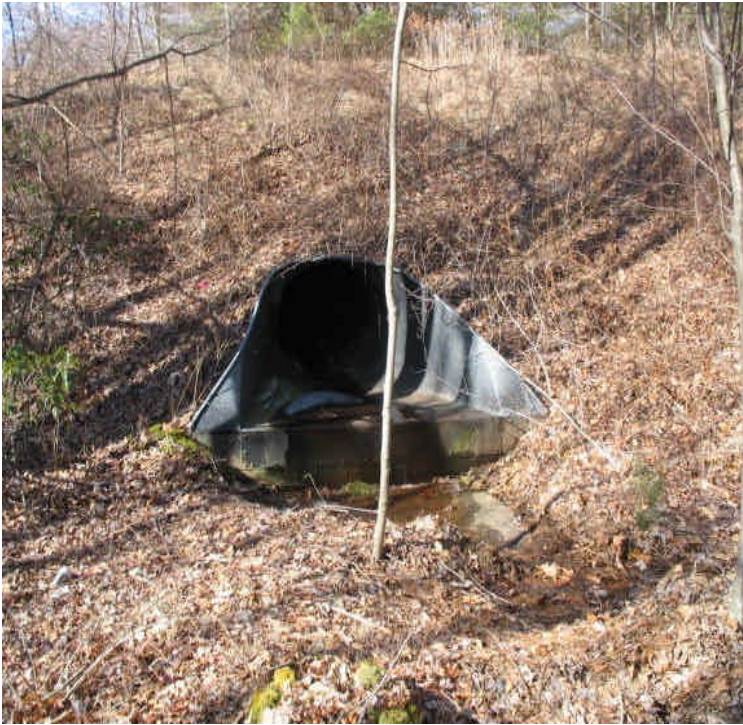
View of the culvert under the access drive. No sediment issues have been observed.
