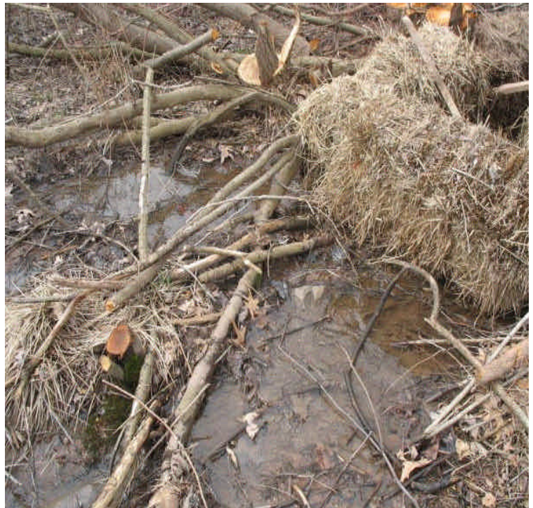
Clear water was observed leaving the haybales and entering the wetland. Evaluate whether the amount of sediment accumulation justifies the minor disturbance needed to remove it, once the water subsides. Timber harvesting/clearing within the wetlands for 2A is complete.
