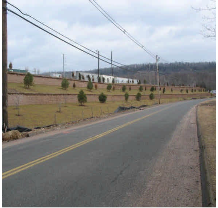
View of Carpenter Lane and retaining walls. Some slight sedimentation (as well as sand from town sanders) was noted along the gutters. Larger piles of sediment have been removed.
