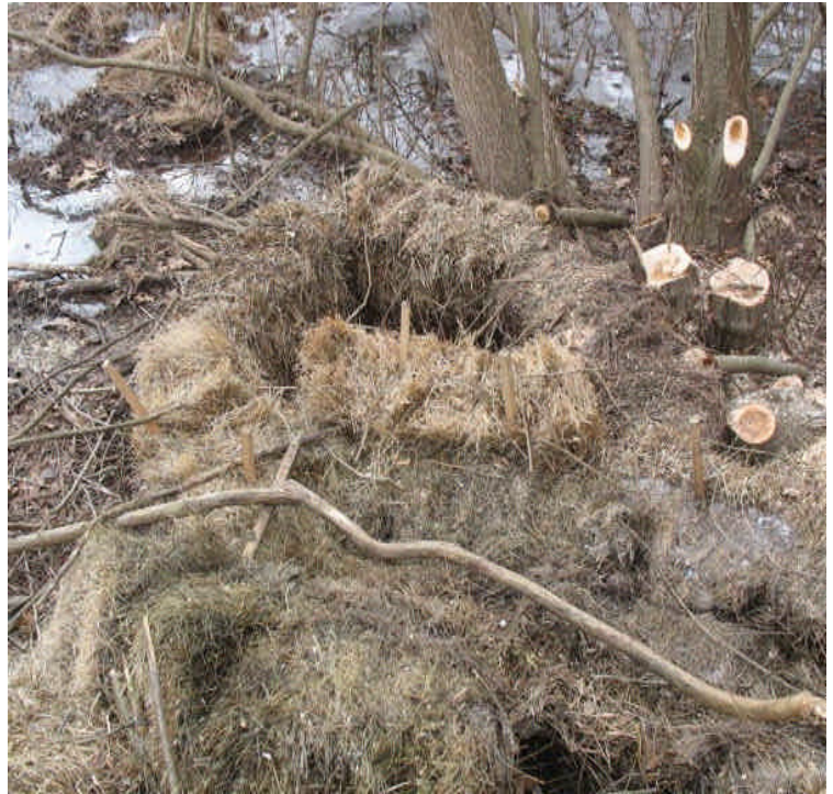
Clear water was observed leaving the haybales and entering the wetlands. Evaluate whether the amount of sediment accumulation justifies the minor disturbance needed to remove it, once the water level subsides. Timber harvesting/clearing underway within wetlands as part of the Segment 2A overhead construction.
