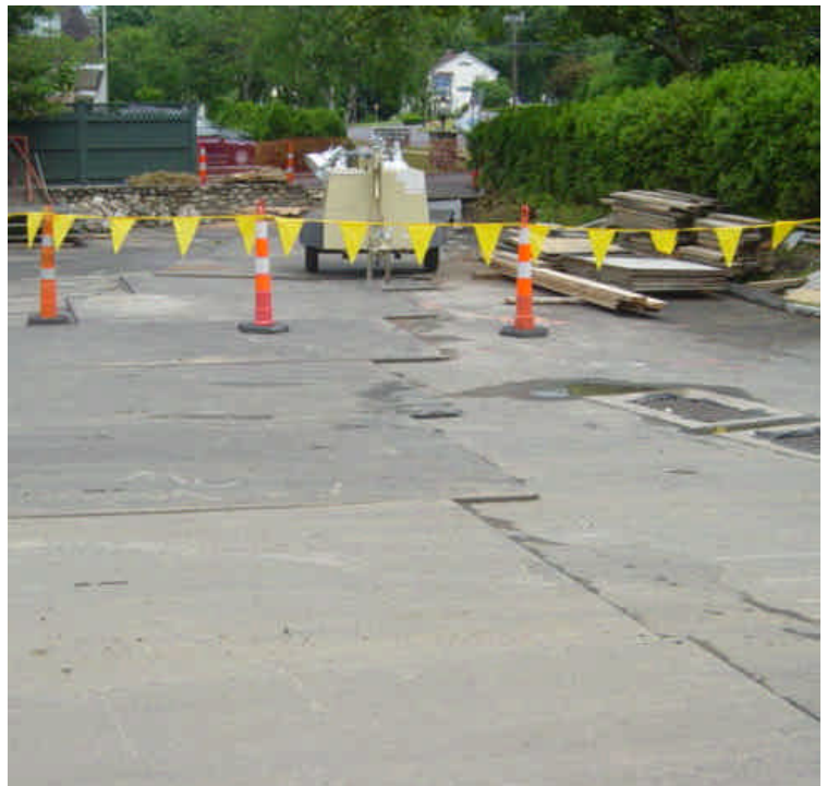
Catch basins located adjacent to sta. #334 were protected with silt sacks.
