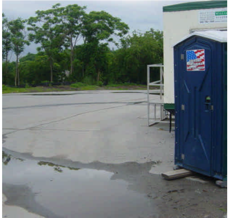
Current condition of the demobilized Imperial Ave. lay-down yard. All that remains is a Sani-can, a construction trailer, and erosion controls.
