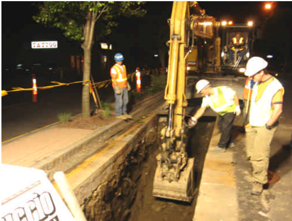
Trenching activities at sta. #698 to #700. Crews had encountered bedrock.
