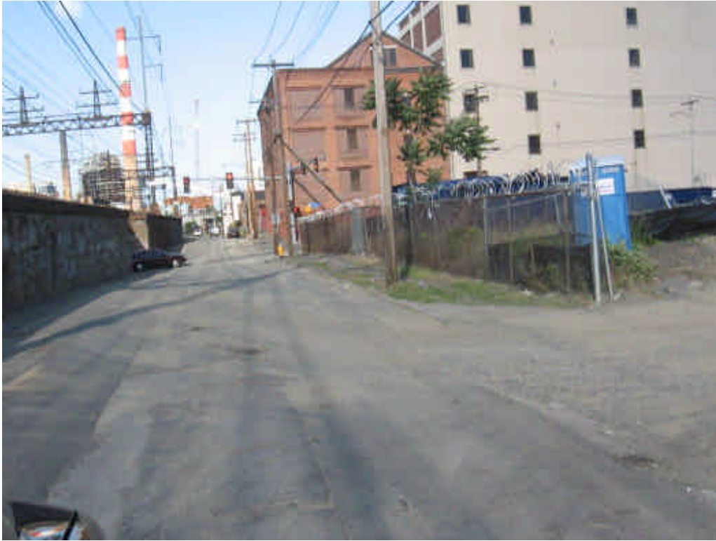
Minimal tracking was noted at Railroad Ave. near its intersection with Myrtle Ave. The tracks were originating from a stockpile yard that is not associated with this project.
