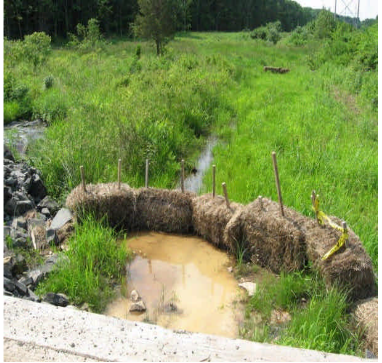
Sediment/turbid run-off was appropriately filtered by a haybale check-dam within wetlands off Carpenter Lane.
