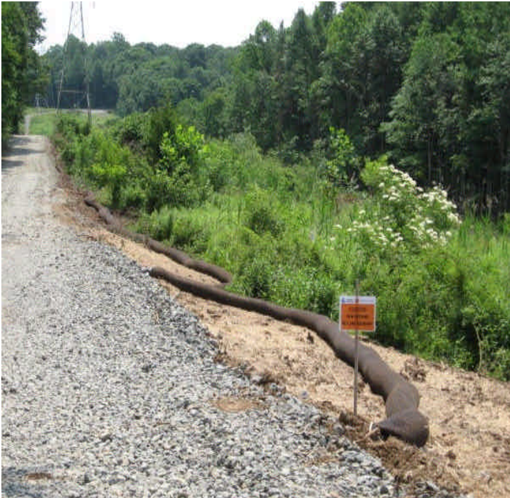
More controls were added upgradient from wetlands off Tuttle Ave.
