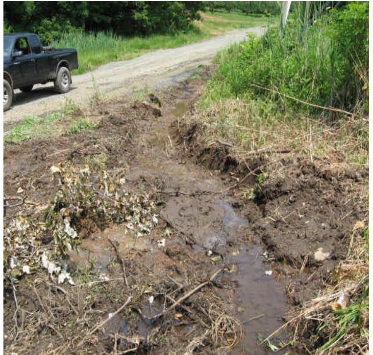
A drainage channel was dug within the apple orchard off Mansion Rd. A culvert appears to be necessary to reduce sedimentation.
