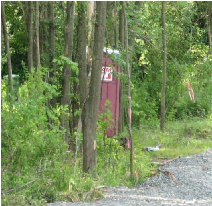
Portable sanitary facility located upgradient from a wetland off Powers Road. Ensure that facilities are placed over 100 feet from wetlands in case of a spill.
