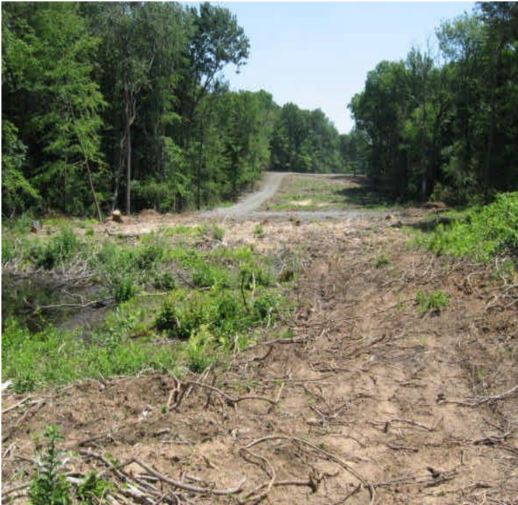
Water was no longer flowing into the pond from the equipment ruts created between Rte 17 and Black Walnut Drive. Controls are still needed. Also, confirm that the “entering wetland” sign is actually at the boundary and not within the wetland.
