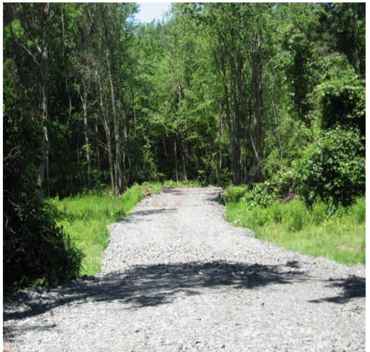
New stone base access road installed near Little Lane.
