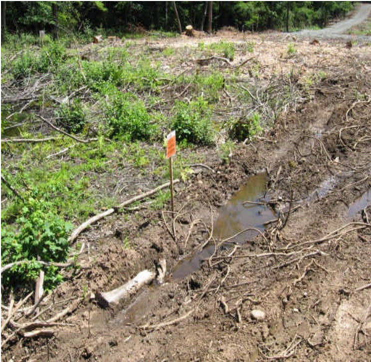
Water was flowing into the pond from the equipment ruts created between Rte 17 and Black Walnut Drive. Access in this area had previously been avoided. Controls are needed. Also, confirm that the “entering wetland” sign is actually at the boundary and not within the wetland.
