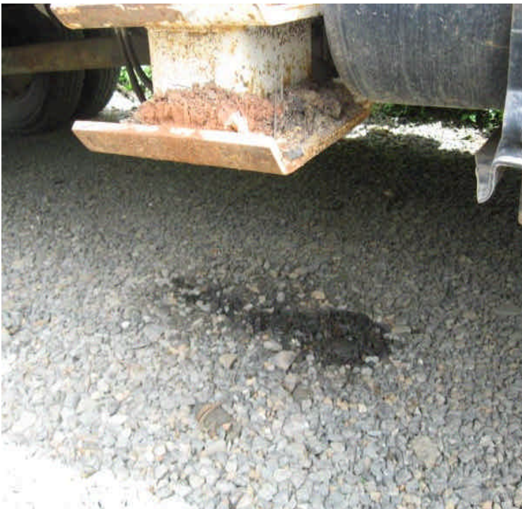
A leaking truck stored within the contractor receiving yard. Several drip spots were noted.
