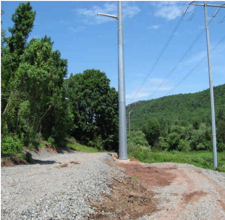
Structure installed north of East Main St, upgradient from a wetland.
