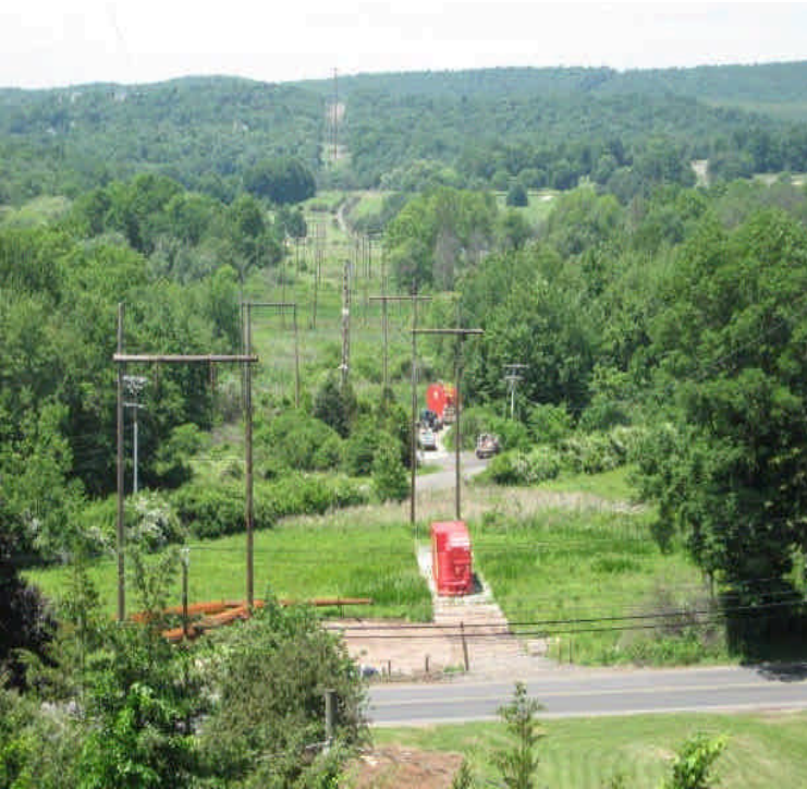
Looking west at Cherry Hill Road & Durham Road work sites.
