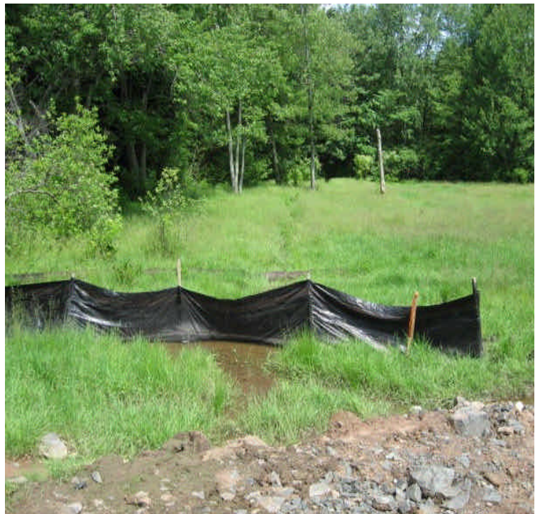
Run-off at the Little Lane wetland crossing. Silt fence check dams were filtering most before it left site.
