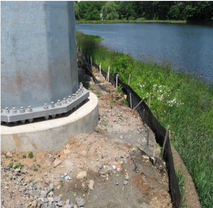
View along the pond north of Beseck SS to E Meriden SS off Fleming Rd where pole installation is complete where sediment has filled controls to capacity immediately adjacent to the pond. A filter sock has been added as another layer of control but sediment should still be removed.
