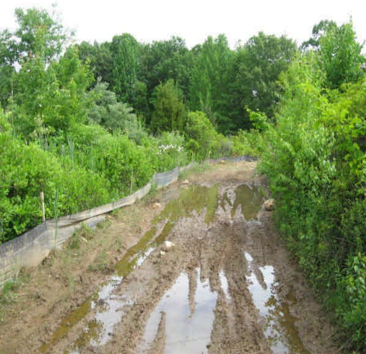
ROW access road south of Scovill SS with ponding water. Controls are in place. ATV use is prevalent here.
