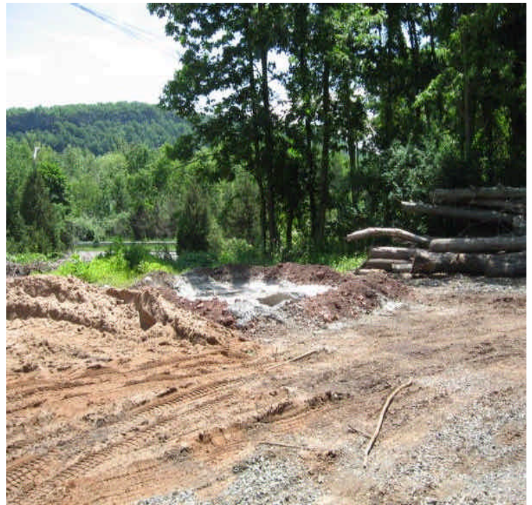
Concrete containment/dump area located north of East Main Street.
