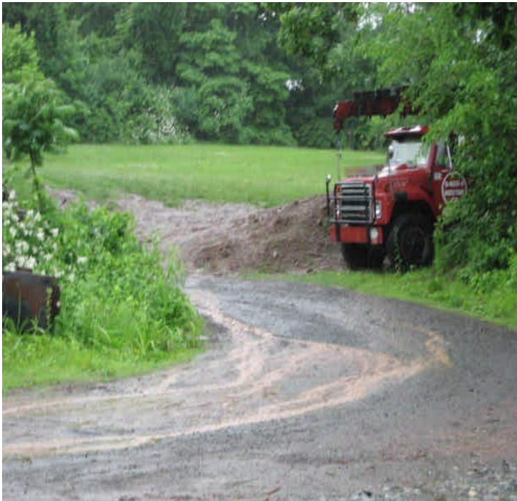
Turbid water flowing from neighbor's driveway/activities and down the access road north of East Main Street.
