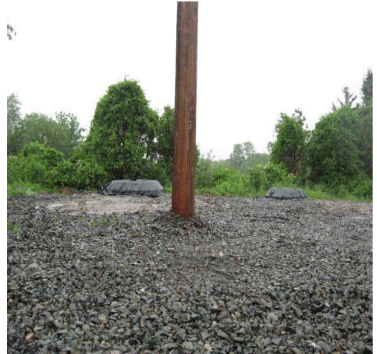
View of new foundations in place at Oxbow Junction.
