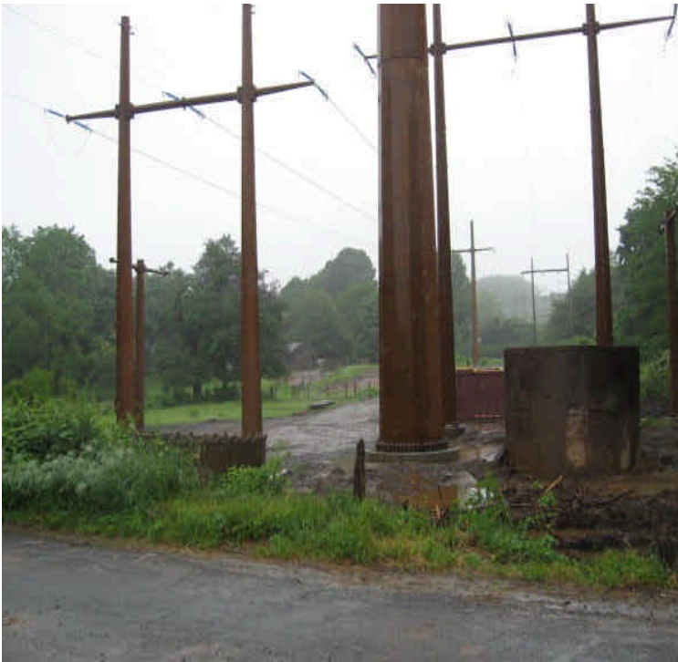
View of structures installed off Little Lane.
