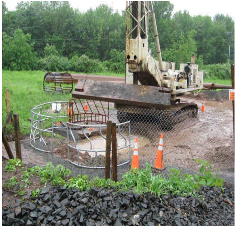
View of a foundation drilled off Cherry Hill Road (west).
