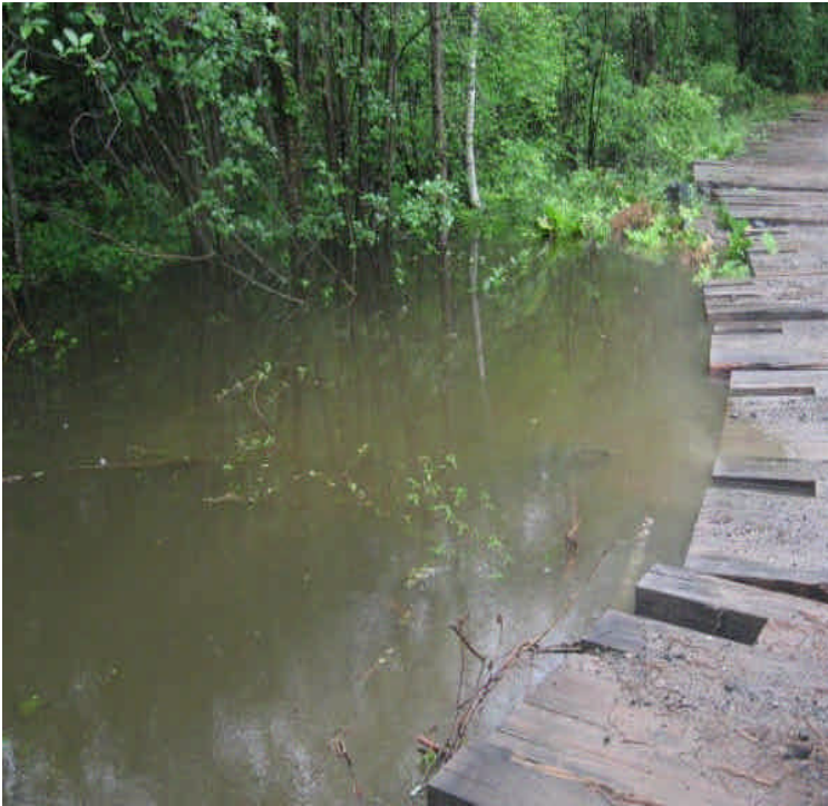
Wetland crossing west of Powder Hill Rd.
