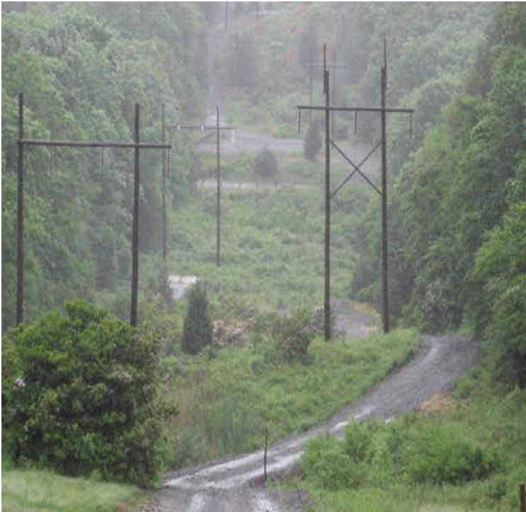
View of the ROW looking toward Foot Hills Rd and Johnson Ln.
