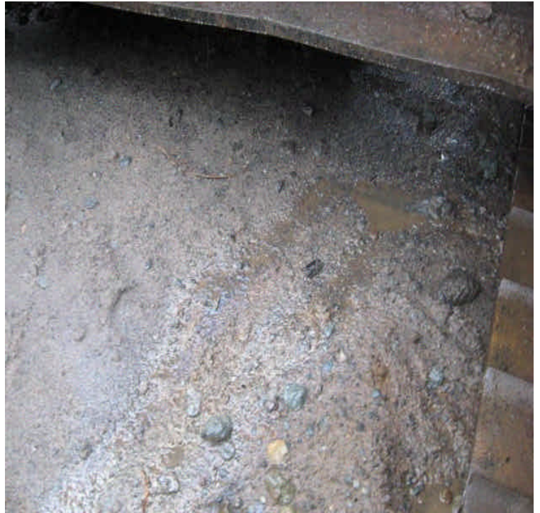
Fluid dripping from a drill rig located off Haddam Quarter Road. Provide maintenance and containment.
