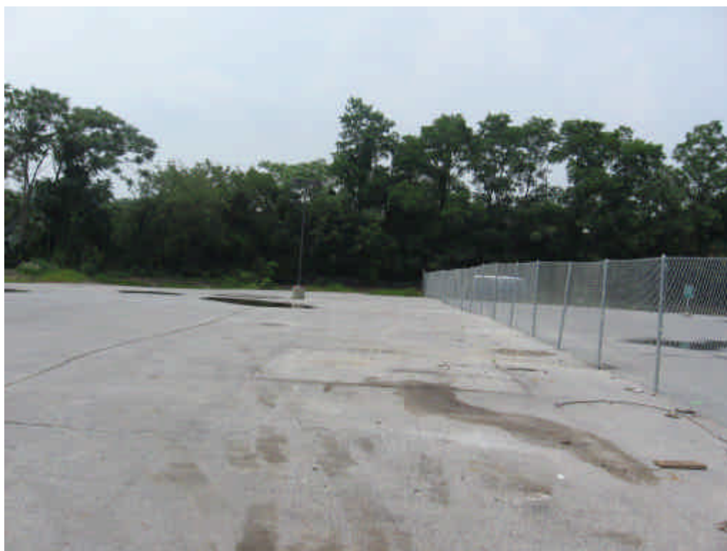
All materials have been removed from the Imperial Ave. lay-down yard in preparation for future staging/bore activities in this location.
