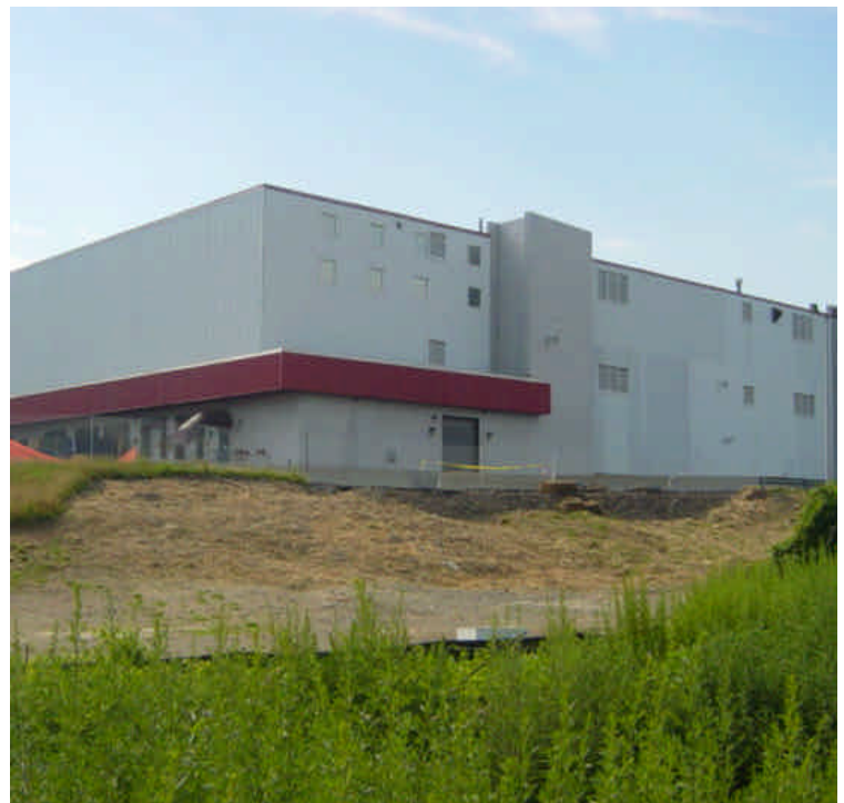
The slope near sta. #1078 has been stabilized with hay mulch.
