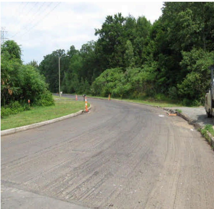
Both photos show the grinding work along Old Farms Rd., in preparation for repaving the roadway and repairing the deteriorating trench patch
