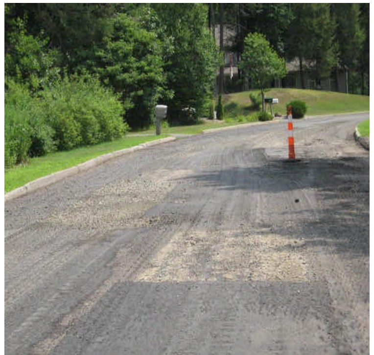
Both photos show the grinding work along Old Farms Rd., in preparation for repaving the roadway and repairing the deteriorating trench patch
