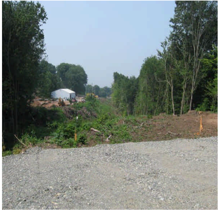
Clearing off Woodhouse Ave looking toward Harrison Rd.
