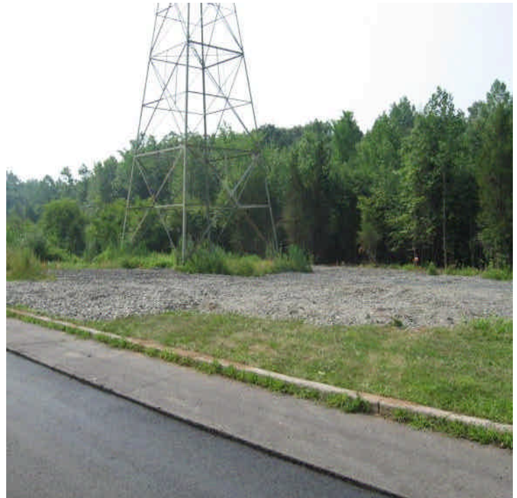
New pad site was installed off Old Farms Road.
