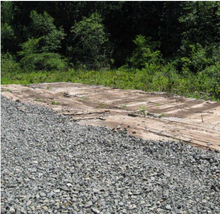
Timber mats installed within the wetlands off Liney Hall Ln.
