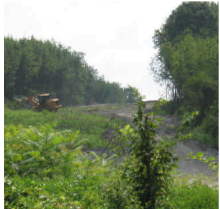
A view of road/pad construction east of Route 17.
