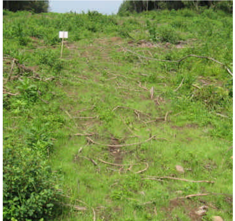
Vegetative growth/cover was starting to fill in where the equipment ruts had been created between Rte 17 and Black Walnut Drive. The area was seeded a few weeks ago. Add controls as needed.
