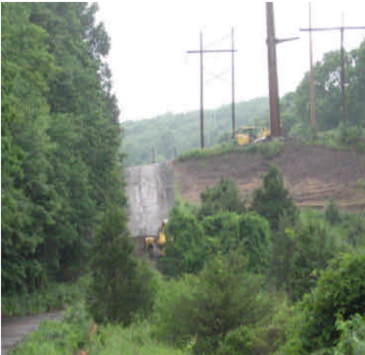
Minor grading activities were occurring off Arbutus Street.
