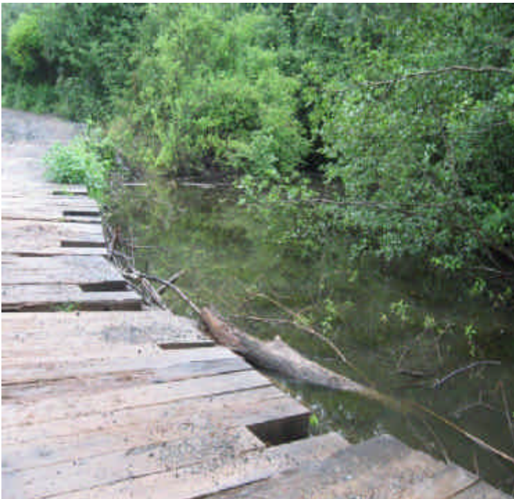
View of the wetland crossing off Powder Hill Rd.
