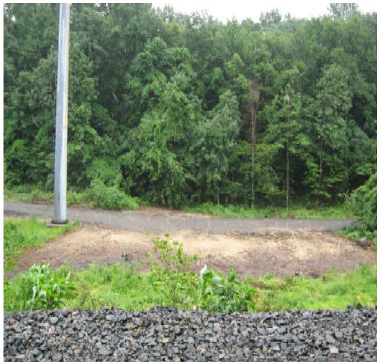
Hay and seed spread to stabilize soils north of High Hill Road along the slope to a stream.
