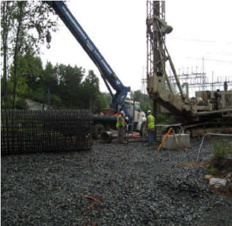
Drilling was occurring west of Scovill SS off Rte 9.
