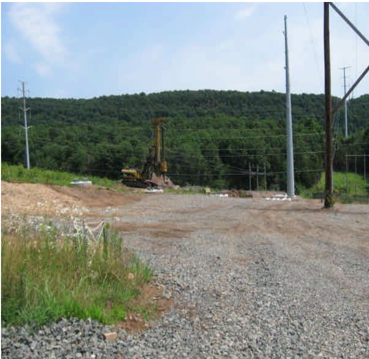
Several foundations were installed north of Beseck SS.
