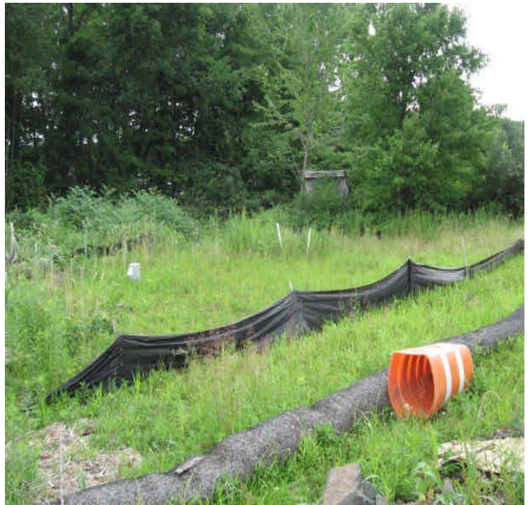
View of the existing controls within the shipping and receiving yard. Repair deteriorating sections as needed.
