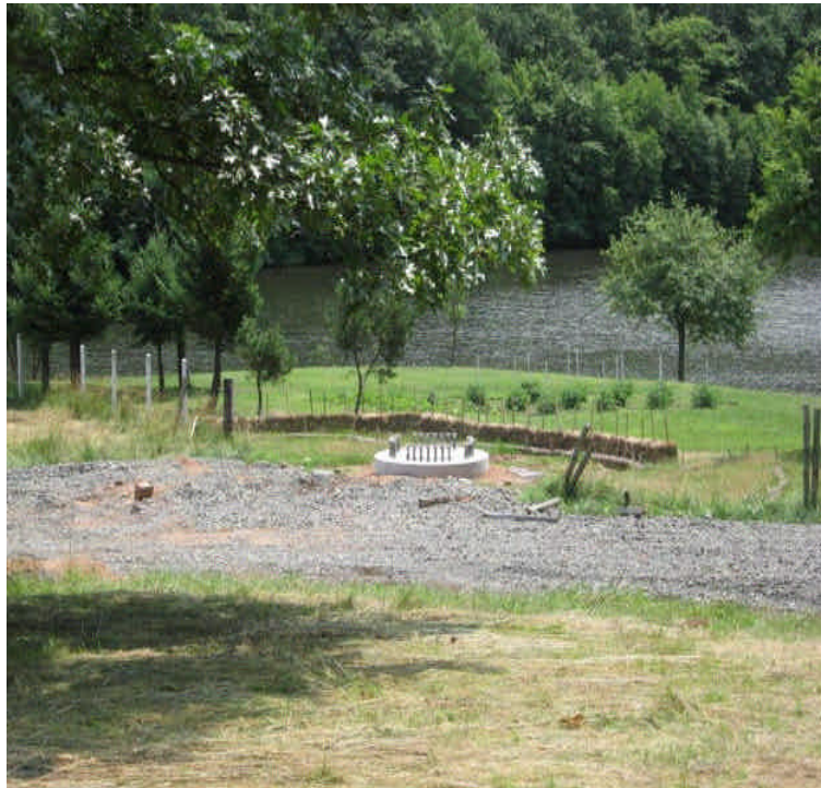
View of the foundation and controls installed off Fleming Road.
