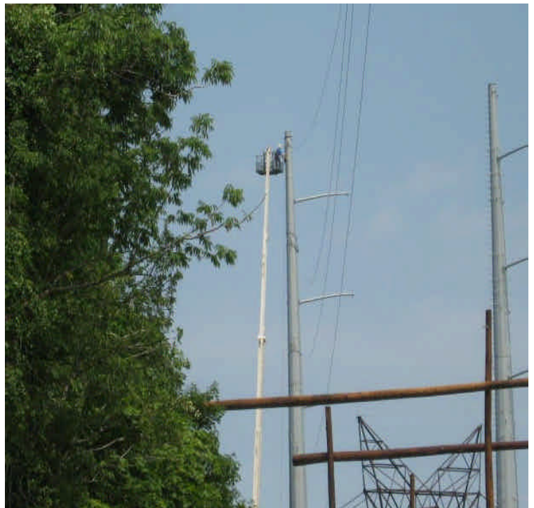
View of the line work occurring at Black Pond Junction.
