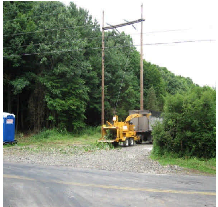
Minor shrub removal and stump grinding/chipping off Arbutus Street
