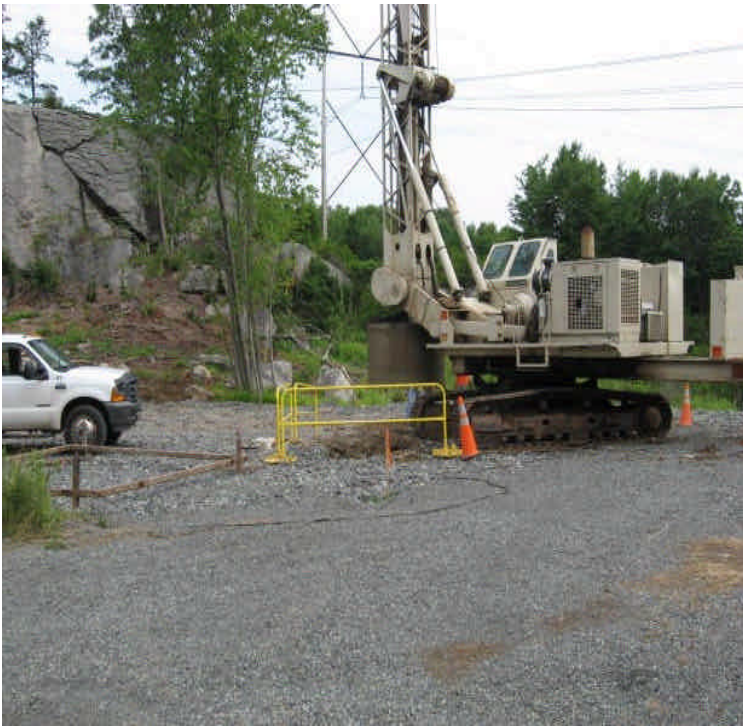
Drilling was occurring west of Scovill SS off Rte 9.
