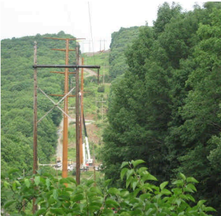
Pole installation was occurring off Johnson Lane.
