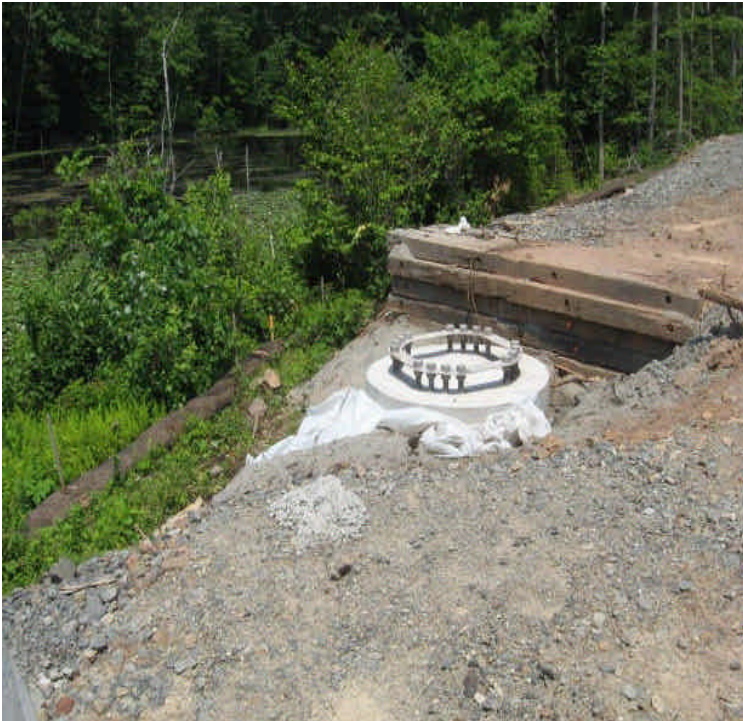
View of the foundation installed west of East Meriden SS.
