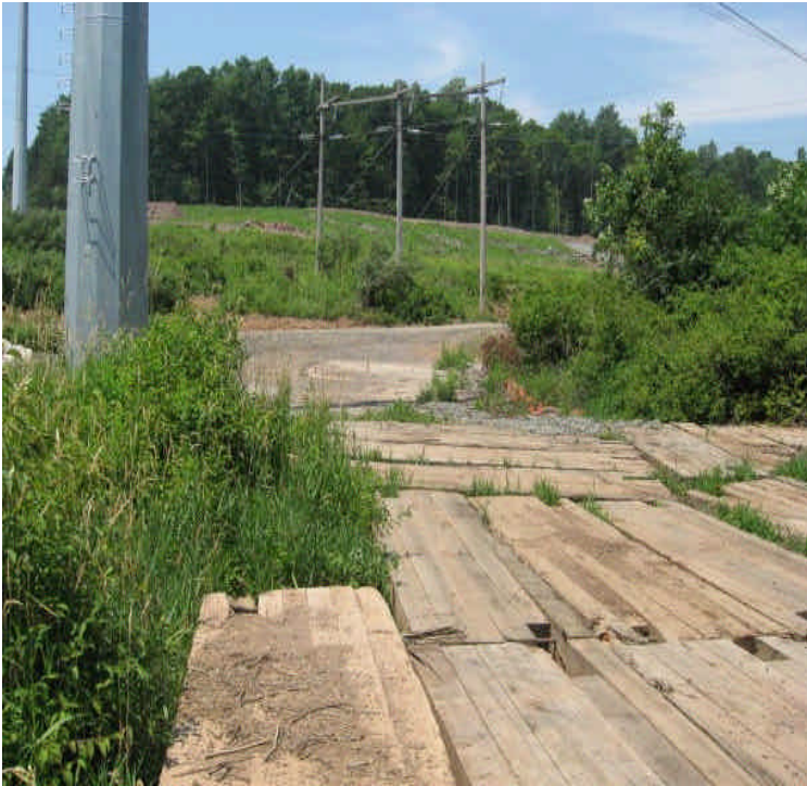
View of timber mats within wetlands east of Beseck SS.
