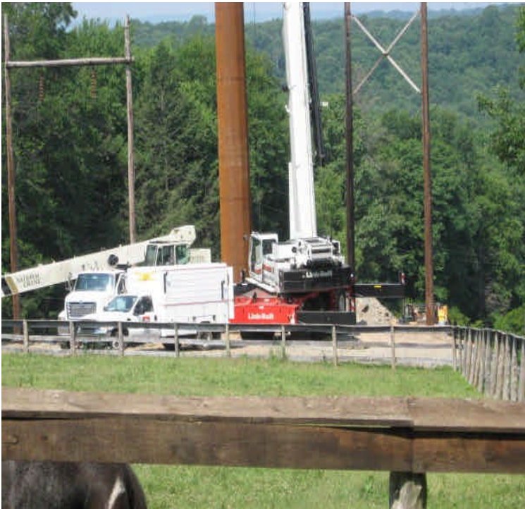
Pole installation was occurring off Foot Hills Rd.
