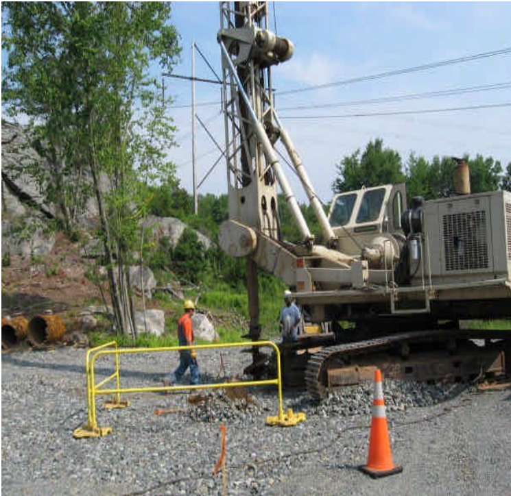
Foundation drilling noted west of Scovill SS off Rte 9.
