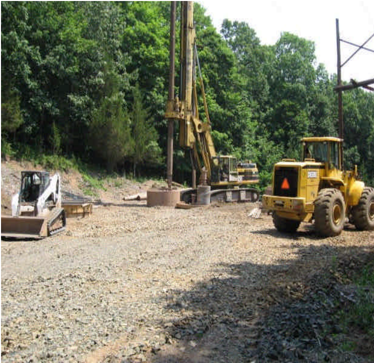
Foundation drilling off Black Walnut Drive upgradient from Ball Brook.
