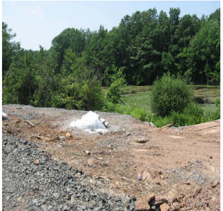
View of another foundation installed west of East Meriden SS.
