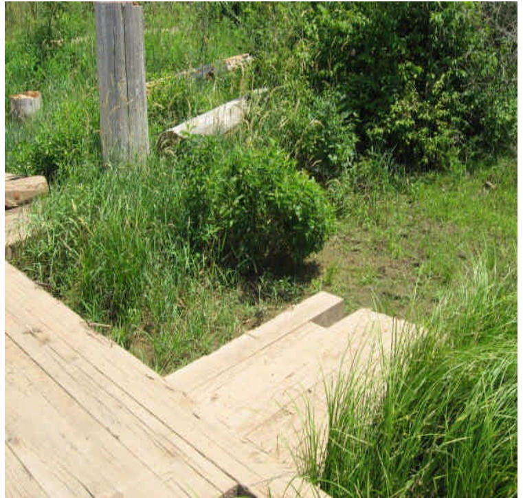
Timber mats within a small pond east of Beseck SS. The pond is dry at this time.
