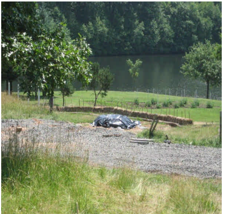
Foundation was installed and controls were in place off Fleming Road
