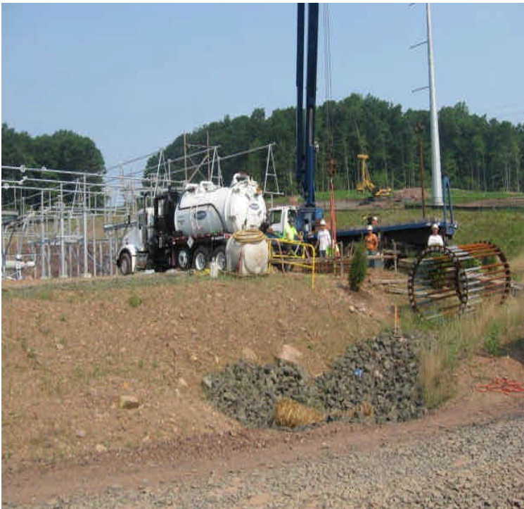
Foundation installation and pump truck at the perimeter of Beseck SS.
