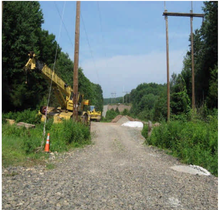
Foundation and pole installation was occurring off Arbutus Street.
