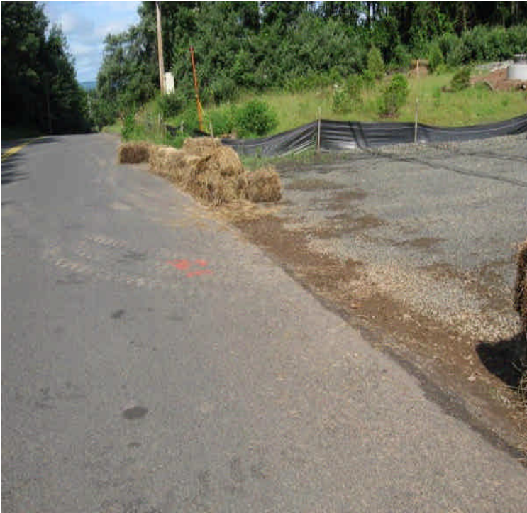
The haybales line was moved from across the site entrance at Carpenter Lane. Restore when feasible.
