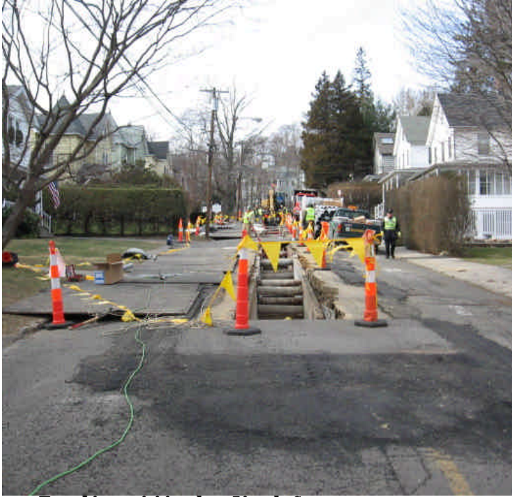
Trenching activities along Lincoln Street.
