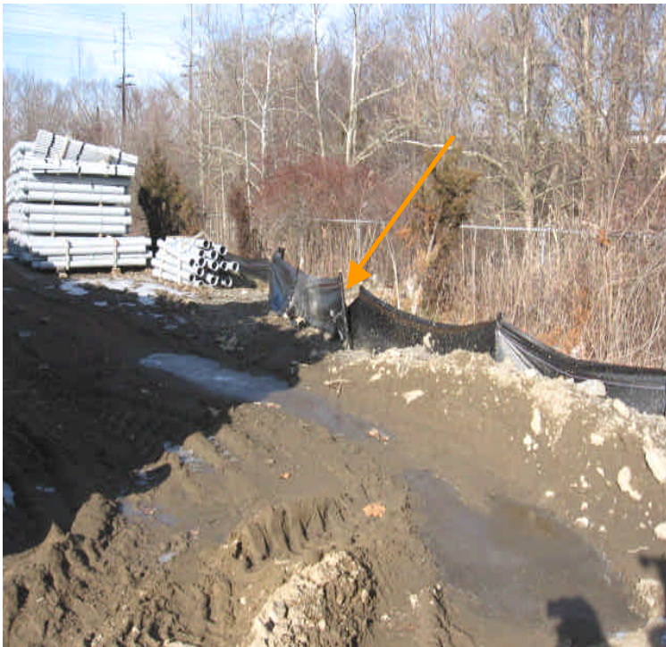
Both photos show the King's Highway lay-down yard. Left: Attempts have been made to repair silt fence; ensure that run-off will not escape at the gaps between sections. Right: Photo of material being removed from yard at the concrete washout basin.
